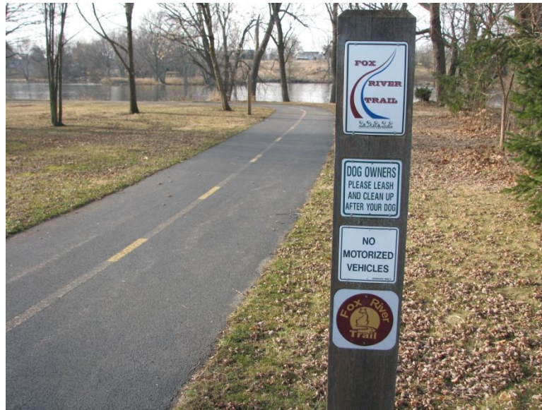
Figure D.44. Typical seal-coated path appearance.
