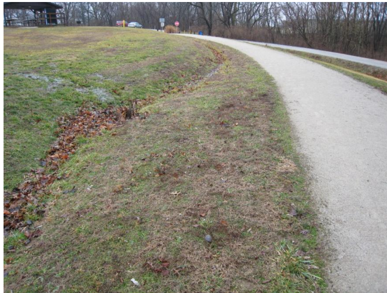
Figure D.9. Adequate shoulders prevent humping, and separation of the trail from drainage components prevents surface degradation.
