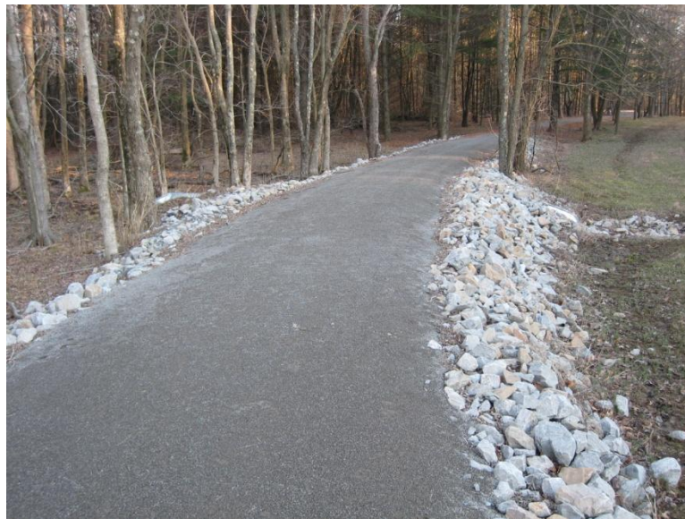
Figure D.21. Fortification of drainage components after installation.
