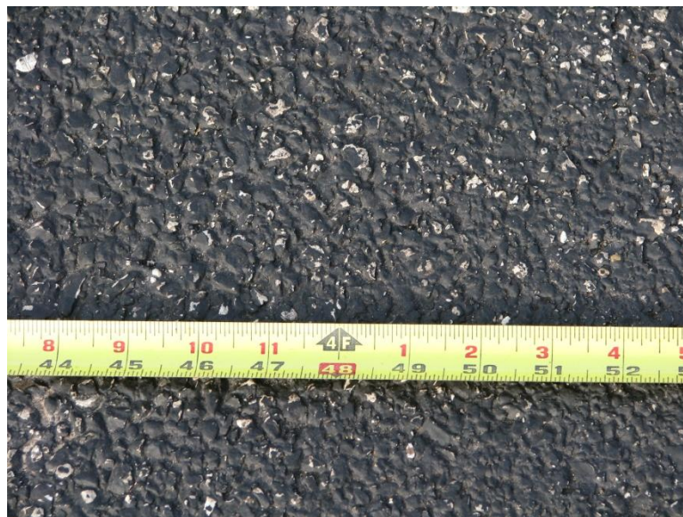
Figure D.45. Seal-coated asphalt trail surface.
