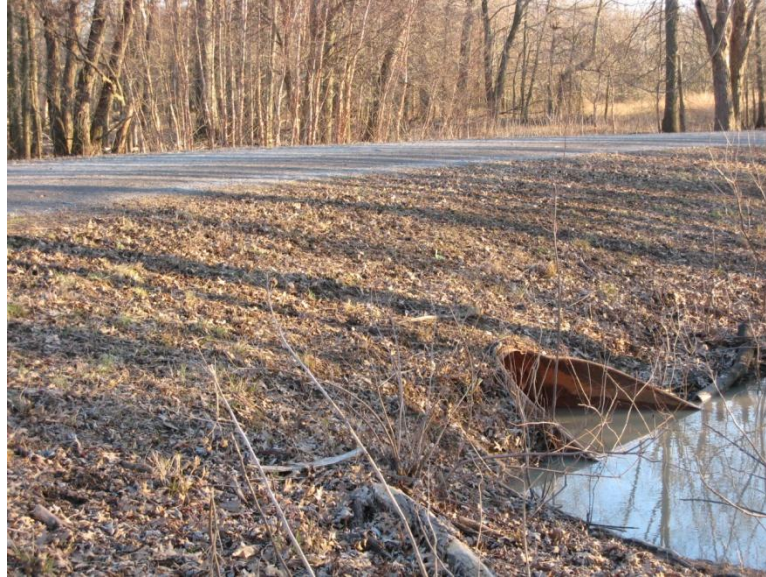
Figure D.18. Good separation between trail surface and culvert.
