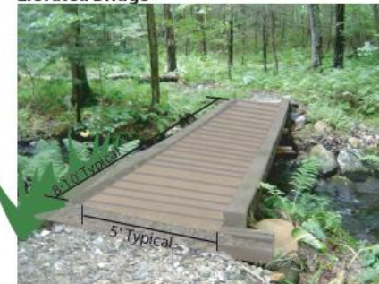
Standard Repair Diagram: Elevated Bridge
