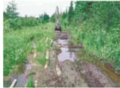
Problem: Compacted and displaced trail in lowland area makes the trail unusable. Altering to drive the trail would cause the entire area unsuitability changing the trail type at an adjacent section. Rerouting or closure of the trail is necessary.
