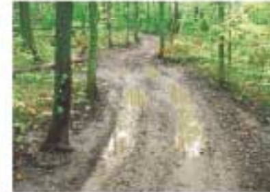
Problem: Compaction and displacement on a new trail site deepening the trail of this relatively new ATV trail. Water runoff will be increased if it is the lowest point. Towing the problem by improving drainage and perhaps hardening the trail through the section are possible solutions.
