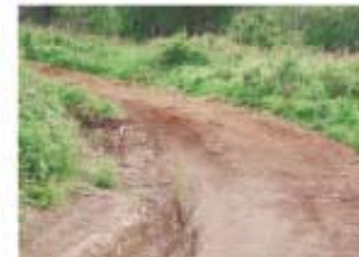
Problem: Severe, ongoing erosion on a roadless slope. Considering the through characteristics of a site is a prescription for the kind of problem. The trail will have to be redesigned using riding grade techniques if it is to be sustainable. Otherwise, closure will ultimately be necessary as the problem gets worse.
