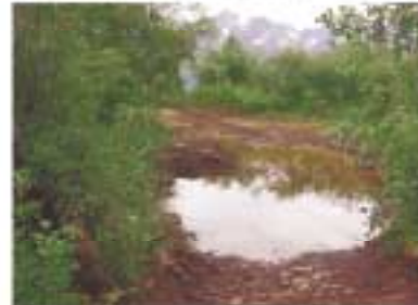
Problem: The ATV trail goes across a shallow drainage that has been deepened through use. This will continue until the hole is too deep to go through. An ATV will have to be driven the area, which will cause further problems. Practice rerouting to the less suitable although closure might be necessary if the problem is persistent in the area.
