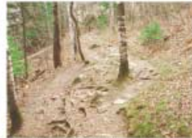
Problem: Exposing trail boundaries. Even a few ruts and ruts in a trail can cause trail users to find another route. Left unchecked, the top of a rut can slowly detach from the trail alignment and the rut will widen. Large gear anchors (and "tree as trail" signs) can be used to keep the flow going west.
