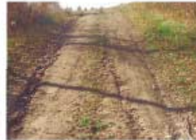
Problem: Erosion due to full-line alignment. In both of these cases, the soil follows the full line (i.e., is aligned straight up the slope), posing an opportunity for erosion. In the left photo, erosion is becoming a problem and soil is eroding to the base of the slope. If geotechnical information is available, the trail could remain temporarily to the left, although a better solution is to regrade. In the right photo, because of a forest canopy, the trail is clearly becoming an issue with increasing use and exposure to the elements. Regrading or closure of the segment will ultimately be necessary to keep the trail sustainable.
