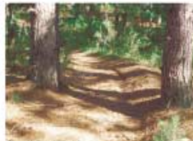
Although the DAM trail is a fairly narrow-use trail, systematic alignment on the curve has formed a superintended curve that allows further displacement. Since the tread remains porous and the site has only gentle slopes, erosion is not a problem and trail is sustainable.
