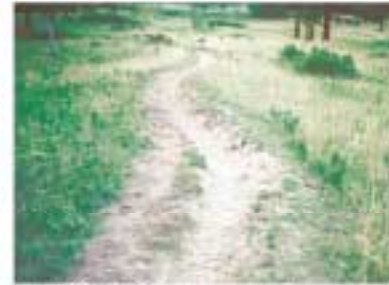
Problem: Soil rutting. With heavy traffic, trail creep can become a sustainability issue. If this is limited to an occasional stretch, no major action is needed. But if this problem persists over a significant distance, regrading or closure may be necessary.
