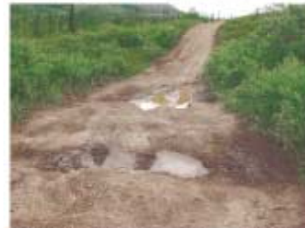
Problem: Trail rutted. If overgrown areas burn and will be left undisturbed, it is a risk that a trail will keep expanding until new options will be created. These problems are common in areas of erosion, with a lot of water there is no real change. Rerouting or practice rerouting to the less suitable. Where that is not possible, consider arguments using riding grade techniques used in a low to deep ruts on the trail can help reduce problems.
