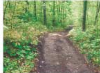
Felling grade design and alignment ensures that the ATP trail will remain sustainable. Careful alignment through dips and crests, erosion can be largely prevented with normal use.
