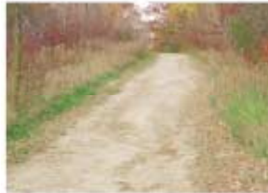
Problem: Erosion due to full-line alignment. In both of these cases, the soil follows the full line (i.e., is aligned straight up the slope), posing an opportunity for erosion. In the left photo, erosion is becoming a problem and soil is eroding to the base of the slope. If geotechnical information is available, the trail could remain temporarily to the left, although a better solution is to regrade. In the right photo, because of a forest canopy, the trail is clearly becoming an issue with increasing use and exposure to the elements. Regrading or closure of the segment will ultimately be necessary to keep the trail sustainable.
