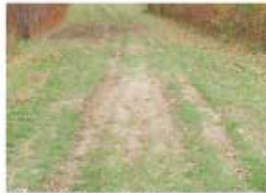
Problem: Lack of underlying soil stability. Organic soils are inherently prone to rutting. Although soil under existing trails, the trail is prone to becoming increasingly unstable, especially if soil height is eroded to adjacent (under) soil water tables. If the soil is too porous, reroading and filling may be the best approach if the problem continues, reroading may be necessary.
