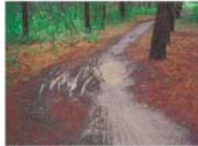
Problem: Trail creep. The low spot on a mountain side trail is gradually widening, forcing trail users to go around it. Careful or removal of the existing path next to a bank that is necessary to avoid additional expansion of the trail.
