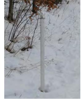
This bollard-mounted light is made of PVC and inserts into a ground socket. It is removed during the off-season.
