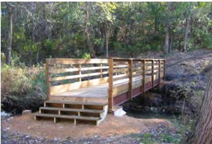
Premanufactured bridges are becoming more popular due to improved materials, aesthetic qualities, and ease of installation. Improvements in design techniques for bridge abutments and foundation systems have also made these appealing.
