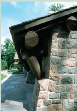
**Flared base.** Walls, piers, abutments, and vertical elements often feel more anchored when they flare outward at the base. A natural example of this is a large tree that flares as it approaches its base. A flared base is an essential design element for trail structures.
