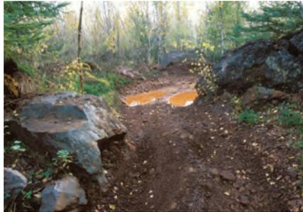
**Challenging mudpits.** When placed at the bottom of a tread climb, mudpits serve to “grease the wheels” and make the climb more difficult. The pit also serves as a sediment trap for runoff from the tread above (left).
