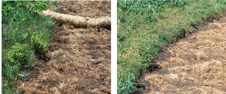
**Good and poor trail blending.** (Left) Since the edges of the rut on this trail were filled to the top, the physical trail scar will largely disappear with revegetation. (Right) With the vertical edges of the trail rut left exposed, this trail tread will remain visible. More fill and/or shaving down the vertical edge is needed to form a gradual edge that would revegetate without leaving a telltale scar.
