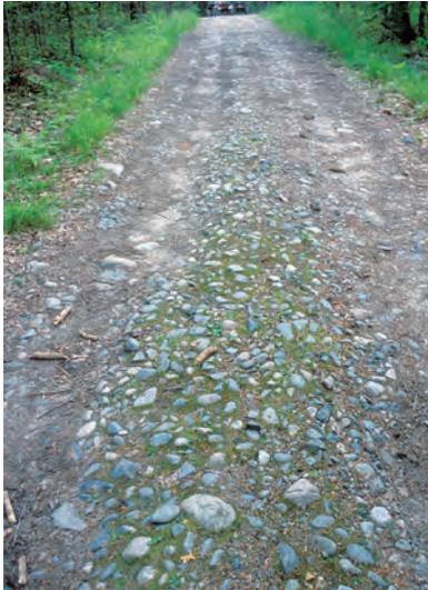
Pit run sand and 2- to 4-inch cobbles were used to harden this forest road segment with an approximately 10% grade. Although ATVs displace some of the smaller cobbles and gravels, larger particles – imbedded in sand and compacted – remain in place.
