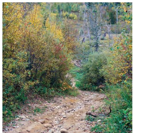
**This eroding forest road in sandy soil drops steeply toward wetlands below.** It is a poorly designed road. Although it could be hardened, rerouting and decommissioning at least this section and forming a new, narrow sustainable trail – or even a new on-road trail to replace the road – may be more beneficial.
