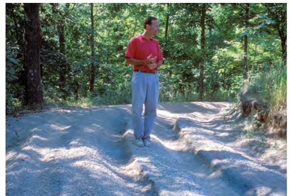
Although crushed limestone can work well for low displacement uses, it is too lightweight and does not contain enough natural lime binders to resist surface displacement by high-displacement uses. Performance in this case could have been improved somewhat by superelevating this curve. (Note that use is already forming superelevation.)
