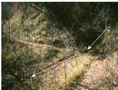
**Correct rolling grade drainage crossing.** The trail crosses this channel in a tread dip. Since this drainage is usually dry and the soil is sandy, water can cross directly on native tread without extensive erosion. The tread climb out of the drainage is visible in both directions.
