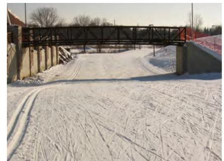
**Combination traditional (classic) and skate style - two direction.** These are generally used as a linear connector between loops or at trailheads where two-direction use is needed. Otherwise, they are not commonly used due to width requirements and the fact that most skiers prefer one direction on busy trails so they encounter fewer skiers. Total width is 16 to 20 feet.
