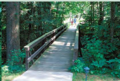
**Contrast of styles.** In many applications, the use of alternative materials has merit to be in sync with the setting. Also, trail widths should be consistent with the intended use. In the left photo, the trail and bridge are 10 feet wide for multiple use. In the right photo, a 6-foot width is appropriate for this pedestrian-only bridge across a small ravine.
