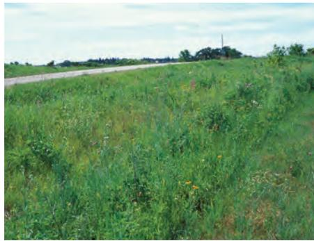
*(Left) The "ribbon infiltration area" between these trails is a depression (about 5 feet deep) to promote natural infiltration of runoff. With native grasses, absorption rates are increased and standing water only occurs after long or heavy periods of rain.*
