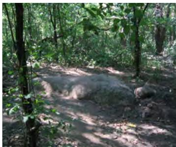
**Boulders for challenge and sustainability.** Vertical climbs using boulders are much more stable than soil-tread climbs. Importantly, these need to be well anchored to prevent bypassing.
