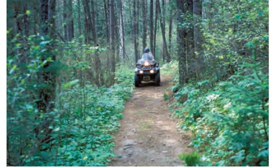
**Hardened logging road with rolling grade.** Overgrown now, this former logging road was partially compacted by logging equipment. ATVs consequently have little effect on the hardened tread.
