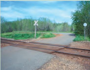
Wood crossings are common in rural settings and work well if maintained. This crossing could be improved by widening it.
