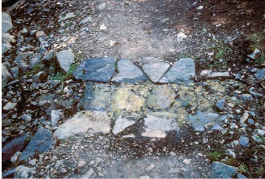
*Hand-fitted stones carry relatively constant spring outflow across the trail. The shallow, ramped dip enables mountain bikes to pass through without muddying the water. This technique is recommended primarily for relatively constant yet low volume flows where water quality is to be protected. Although installation is labor intensive and requires a supply of stones with flat faces, the result can be an attractive trail feature that accentuates the water passing through it.*
