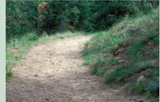
**Additional tread width.** The tread is 8 to 42 inches wider than it would be on a lesser sideslope. This is often useful on limited sightline or blind curves with an outside drop-off. The outside edge is not initially raised but may become bermed as the center is compacted and displaced material mounds on the widened edge.
