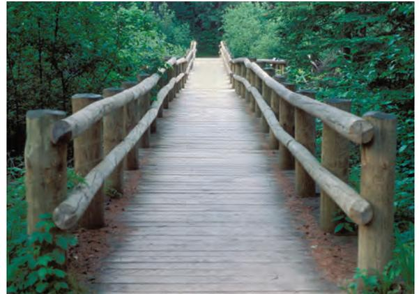
*Thick timber posts, thinner rails, nonsquare ends of posts and rails, and overlapping joints are rustic elements of this pedestrian bridge. The objective of rustic structures is to create a relaxed, natural character by avoiding straight or curvilinear lines, allowing rough materials to shape the details of how parts fit together.*
