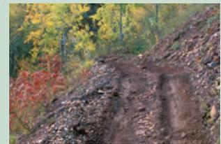
**Inslope.** A narrow tread can be shaped to slope and drain to the inside edge. If trail users start to slide sideways on a loose or slippery tread, they will then slide inward, away from the edge. Rolling grade is used to drain the tread. Inslope is often combined with a bermed outside edge.
