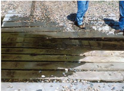
**Concrete boat ramp planks.** Planks laid on aggregate fill can provide lateral stability for slow water crossings. Planks are laid perpendicular to the trail.
