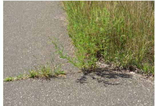
*This trail, which is also only three or four years old, is showing the impact of prairie grasses and weeds growing in pavement cracks. Keeping the shoulder mowed and filling cracks each year is a reasonable and cost-effective solution here, rather than using a root barrier.*
