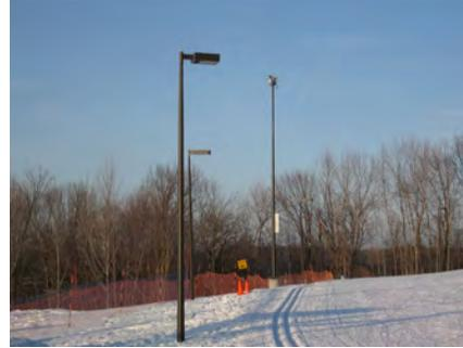
A down-facing box light is also occasionally used on ski trails, although the lighting is more apparent. This type of fixture is more commonly used at trailheads, where a larger pool of light is desired.
