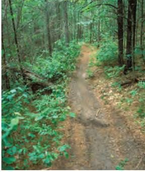
This OHM trail is at least 25 years old and has had virtually no maintenance. Rolling grade, coupled with gentle grades and the tree canopy, prevent erosion. The sandy loam tread absorbs much of the runoff, along with well-placed tread dips draining the rest.
