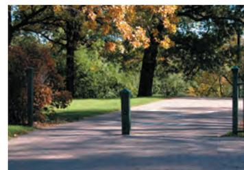
Bollards are commonly used to deter motorists from accessing trails. Typically, bollards are set 48 to 60 inches apart when across a trail, often with the center bollard being removable for authorized vehicles.
