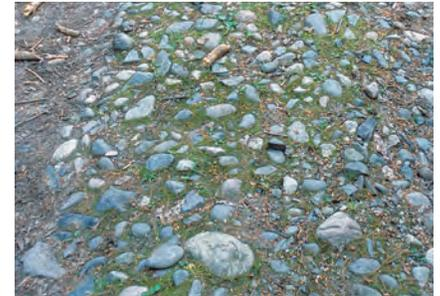
Mechanically stabilized rock and soil-hardening techniques are often used for drainage crossings.
