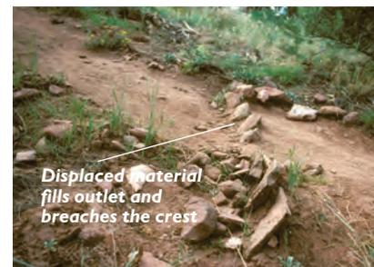
Doomed from the start, this very steep tread grade is close to the fall line. With a very narrow outlet, the waterbar slows water coming down the tread and acts as a settling point for displaced tread material, which breaches the crest.
