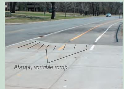
**Abrupt pavement changes can catch trail users off guard.** Although difficult to see in the photo, the ramp is uneven and short. This can cause bicyclists and in-line skaters to drift out of their lane into oncoming traffic.
