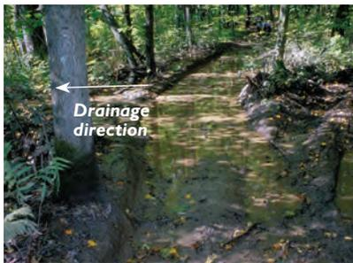
High displacement and insufficient sideslope have allowed compaction and displacement to lower the bottom of the dip below the bottom of the outlet, ponding water in the dip.
