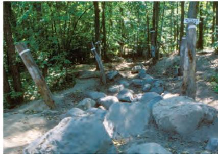
**A rock-pile obstacle** provides a challenge that is well anchored by trees and larger rocks, minimizing the chance to go around.
