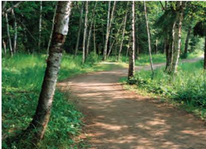
**Crushed stone.** In this nearly level site for a multiuse trail, native soil was replaced with crushed stone. The tread surface is only slightly raised above the surrounding ground.
