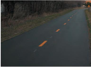
*This trail was sealcoated with a black sealcoat with no sand or crushed rock chips, which makes for a smooth surface, although a bit more slippery than asphalt. For many, the value of sealcoating remains uncertain.*
