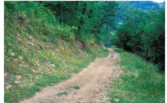
**Excellent sustainability.** This portion of the Southeast Minnesota ATV Trail – a trail conversion – has rolling grade and excellent drainage to the side. Note the steepness of the sideslope – up to about 70 percent slope.
