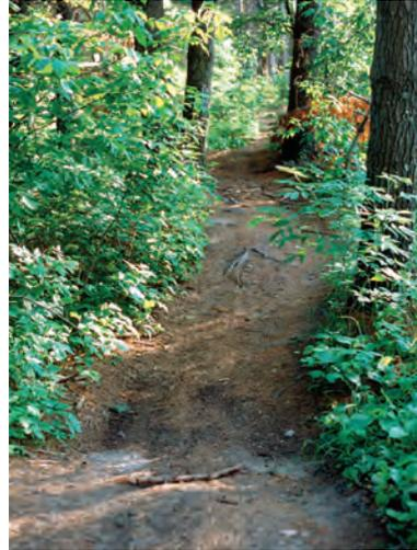
*Both of these trails are well-anchored to keep mountain bikers (left photo) and ATVs (right photo) on the trail through an alignment dip. Note the small superelevation on the mountain bike trail, which does not clog due to enough fall-out from the dip and routine maintenance.*
