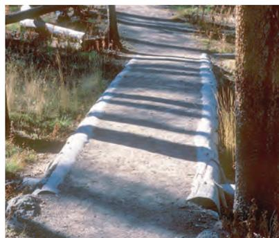
Turnpike can be used to form a raised approach in areas of unstable soils. A timber or conventional culvert can convey water under the structure, or a paved dip can carry water through it. In a near-level drainage crossing with boggy soils, ditches may need to be dug on both sides to lower the local water table below the level of the logs.
