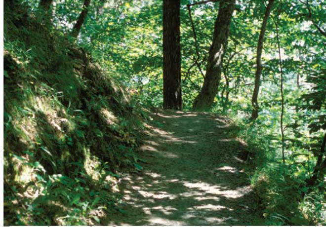
**Topography as anchor.** Cutting a trail into a sideslope firmly anchors the trail in three-dimensional space. The sideslope also provides the visual connection to the next anchor, which is the tree that forces a change in direction. As the cutslope and fillslope revegetate, the trail will seem like it has always been here.
