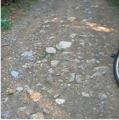
Rocky soils make some of the most durable treads. The cohesive structure distributes weight and functions equally well wet or dry. Rock size, however, needs to be matched to the type of use or visitors will tend to go around, rather than over, the rocks.
