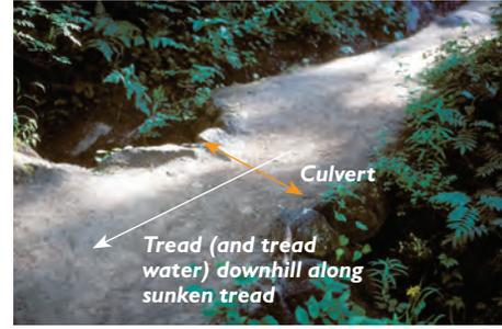
**AVOID where possible.** Although very nicely formed with stone headwalls and tailwalls, if this deep-channeled culvert were to clog, water would be diverted down the tread because there is no tread dip. Also note how tread wear has depressed the center of the tread, allowing tread water to follow the tread over the culvert.
