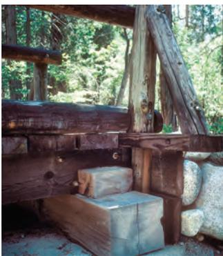
The timber sill on this stone foundation has a mortared cap. The end cap extends behind the sill to protect it from soil contact. The wide endcap and stones harden the edge and help retain the trailbed.
