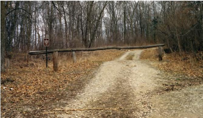
A trail closed with a gate remains inviting to use, and the gate, even when combined with fencing, is often bypassed. Although gates are commonly used for seasonal closures, they are not typically enough to formally decommission a trail.
