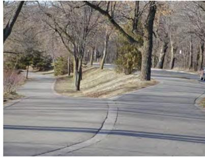
**Separated and directional trails.** The trail farthest to the left on this photo is for two-way walking and jogging. The trail to the right is a one-way trail for bicycles and in-line skaters. The one-way trail works in this situation because the trail loops around an urban lake. The high use volumes justify the 10-foot width for both trails. The green boulevard between the trails adds to the character of the trails and helps reduce conflicts between users.
