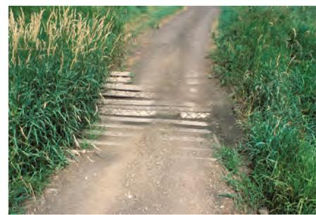
**Paved dip for ATVs.** Small concrete planks have diagonally scored faces for traction. Since this is a low flow, seasonally flowing drainage, planks are set directly in native soil tread.
