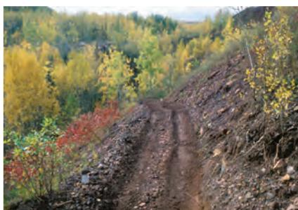
**Exposure creates drama.** Sideslope trail alignment creates an increasingly dramatic feeling of exposure as the sideslope increases. At the same time, alignment on steeper sideslopes maximizes tread drainage and physical sustainability (left).
