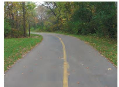
A solid yellow line is used to identify a no-passing area when approaching a curve or hill with limited sightlines. This is often accommodated with a trailside warning sign.
