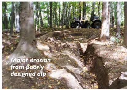
The lack of a well-designed rolling grade on this ATV trail has resulted in too much water flowing through a dip and creating a major erosion problem that is not sustainable. This trail will have to be redesigned.
