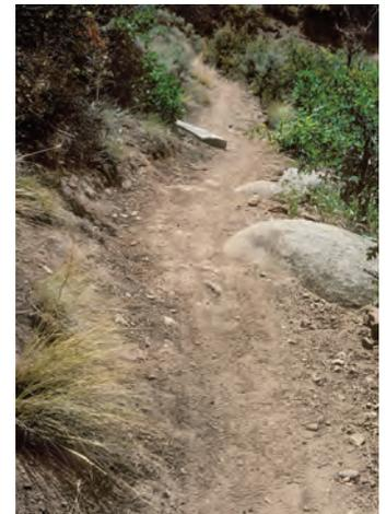
*The large natural stone anchors and also forms this in-line alignment crest. Stones can also be placed in trails with heavy equipment, especially where a roadway tread is being narrowed in a trail conversion.*
