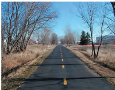
On this regional level trail on a rail grade with long sight lines, a 20 mph travel speed would not be uncommon – faster on downslopes and with a tail wind. Although the trail can accommodate the speed, above 20 mph trail conflicts can become more likely.
