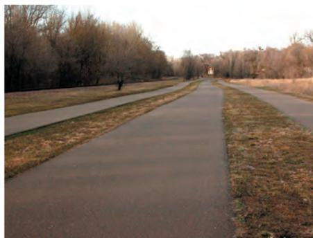
(Left) Although not really noticeable to the trail user, this trail is perched high enough to consistently drain into adjoining natural areas, where water can percolate into the ground.
