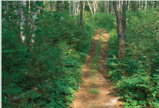
In undulating terrain, short fall-line climbs can be sustainable. In this example, a gentle tread grade, gravelly and well-drained sandy loam tread, tree canopy, and low use all help protect the tread from displacement and erosion.
