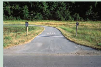
**Curve sets up a crossing.** This easily visible curve slows trail users down as they approach a road. The open sightlines ensure that the curve and crossing can be seen in more than adequate time for the trail user to slow down and stop.
