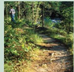
*Compaction and erosion leave rocks and roots protruding from an otherwise smooth trail.*
