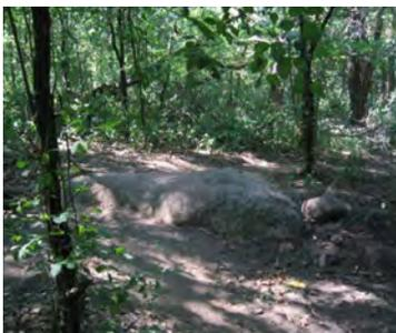
**Boulders for challenge and sustainability.** Vertical climbs using boulders are much more stable than soil-tread climbs. Importantly, these need to be well anchored to prevent bypassing.
