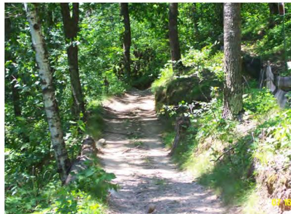
*(Right) Trees and a sideslope help anchor this crest (top of photo) and dip bottom of photo) along an ATV trail.*
