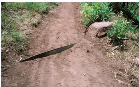
(Upper left) A 30 percent tread grade needs higher maintenance. The bar is silted in and partially collapsed on the outsloped tread for mountain bikes. The bar is also too short on the right side.
