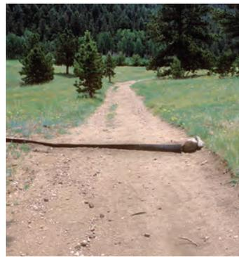
This tread runs near the fall line, with a sideslope down to the left. The bar uses outside slope on the tread to accelerate water to the dip. Notice from the small gullies in the left foreground that most water never reaches the actual bar.
