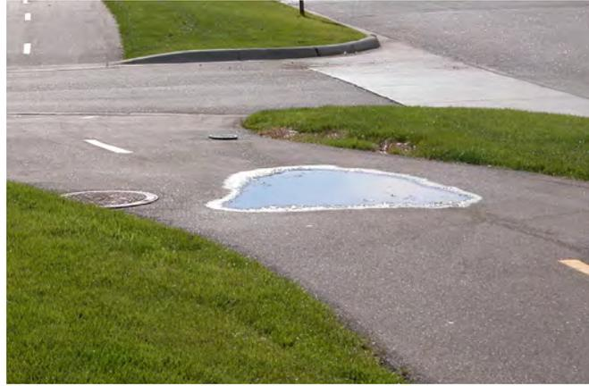
"Bird baths" are largely avoidable if the contractor is paying attention to subgrade preparation and cross slope prior to laying down the pavement. This dip should be corrected.
