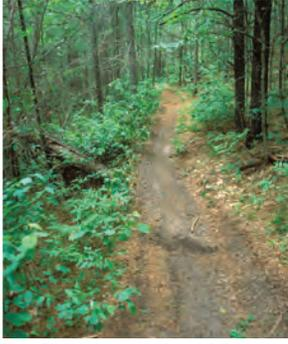
This OHM trail is at least 25 years old and has had virtually no maintenance. Rolling grade, coupled with gentle grades and the tree canopy, prevent erosion. The sandy loam tread absorbs much of the runoff, along with well-placed tread dips draining the rest.
