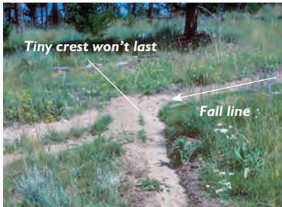
Outlet decelerates water and is too narrow, causing sediment buildup. The dip outlet should follow the fall line to move water away from the trail faster. The sandy tread is also unstable, which suggests a need for more crests and dips.
