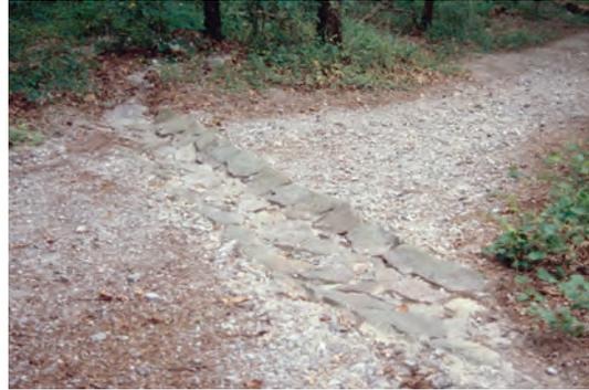
Where there is little sideslope, the stone paving should extend beyond the tread on both sides to ensure full coverage. Attractive stone paving is considered a desirable feature on nonmotorized trails, especially hiking trails. Using a variety of stone shapes adds natural shape and enhances rustic appearance.
