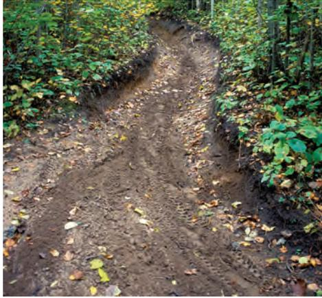
**Problem: Excessive displacement.** Heavy use, erodible soils, and lack of rolling grade have combined to excessively displace soils along this trail. Rerouting and/or closure is necessary since fixing this is almost impossible.
