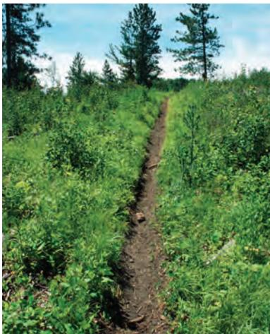
**Tomorrow's problem!** *While this new OHM tread may seem sustainable today, it has already compacted and displaced into a trench. Since it runs directly up the fall line of this slope, it will soon erode as water follows the tread straight downhill. After only one year, erosion has already begun, with the bottom of the tread being deeper than the top.*
