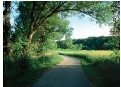
This is a typical **city or county trail** through an established greenway corridor. A 10-foot width is optimal on most trails, but 12-foot widths are also used in very heavy use areas.
