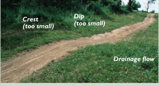
**Partial implementation.** This filled crest is working for now, partly due to very stable tread soil. The crest, however, has little effective volume and the dip is very shallow. In sandy soil, displacement would quickly wear the crest down and sediment would likely clog the dip.
