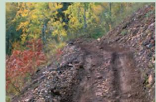
**Inslope.** A narrow tread can be shaped to slope and drain to the inside edge. If trail users start to slide sideways on a loose or slippery tread, they will then slide inward, away from the edge. Rolling grade is used to drain the tread. Inslope is often combined with a bermed outside edge.
