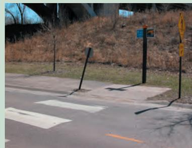
This is simply a poorly placed ramp and signage combination. The sign is a hazard and the ramp is too small and abrupt to be of much value to trail users, especially bicyclists.
