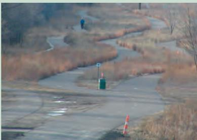
**Curves used to slow down traffic.** As these trails converge into a narrow corridor under a bridge, curves and visual cues were added to slow down bicycle traffic. The long, open sightlines make this approach suitable for this situation.
