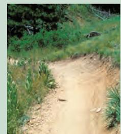
*This superelevated curve resists horizontal displacement while draining well.*
