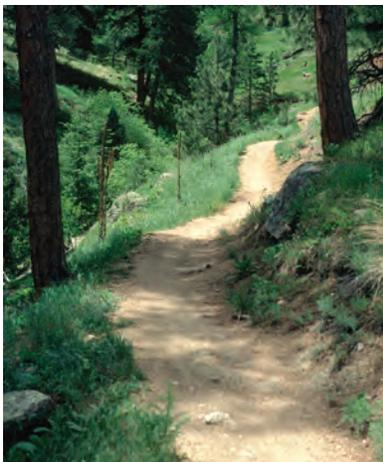
**Ideal rolling grade.** Crests and dips are formed through tread alignment. Compacted through trail use, this tread is stable enough to resist displacement in most places. Steep slopes above the trail (to right) pour large volumes of runoff onto the tread, but the tread handles it with gentle grades and small tread watersheds.
