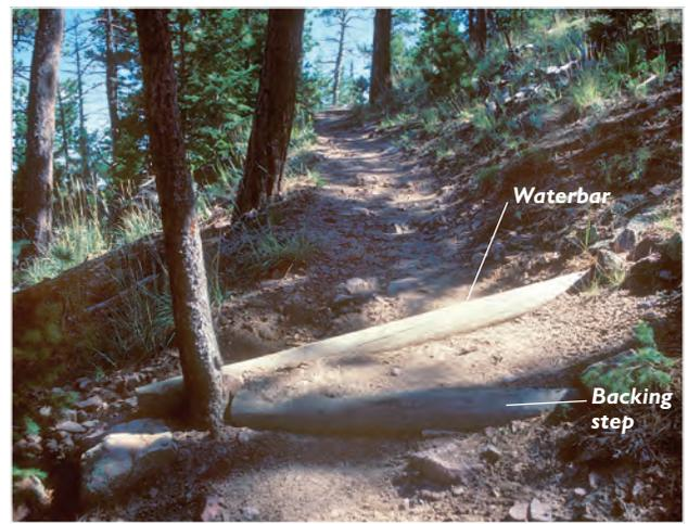
A backed waterbar is sometimes necessary on steeper tread grades. It also makes for a comfortable step in the ramp behind the bar while it stabilizes the ramp. This is typically built as a riser perpendicular to the tread. Note how this waterbar is anchored on the tree at left.
