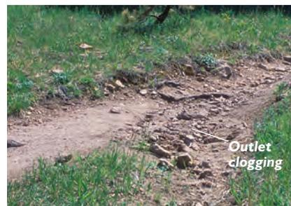
This outlet was clogged by dry displacement that settles in the dip through everyday trail use. The tread grade is approaching the fall-line, further exacerbating clogging.
