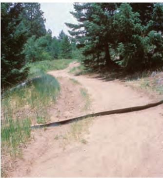
The angle of this bar was reduced due to high outside slope on this superelevated curve. As long as the water runs off at as steep a grade as possible, the bar can be placed more perpendicular to the tread.
