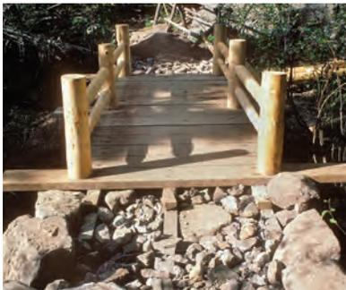
Seen under construction, the ends of three steel stringers (topped by wood nailing strips) are embedded in this un-mortared stone abutment. Stone minimizes the footprint of the raised abutment while visually anchoring it. Rock fill provides excellent drainage and reduces settling and tread displacement.
