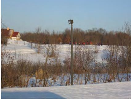
The common pole-mounted high-pressure sodium fixture faces down the trail in the direction of travel to avoid putting light in the face of the skier and night ski. With buried wire, a natural-colored pole, and a small fixture, the light serves its purpose with minimal visual intrusion.
