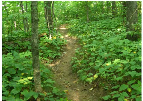
**This sustainably designed trail naturally follows site contours**, which also make the trail more appealing. Notice the trail drainage dip that drains water off the trail (to the left).
