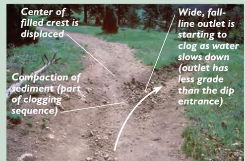
Although this deeper dip and crest are working for now, they need repair and cleanout. The deep dip is filling with displaced tread material because its outlet is less steep than the tread above it. The crest (which lacks effective volume) is also losing its center through displacement, mostly by mountain bikes.
