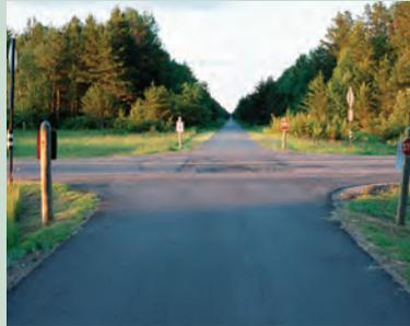
**Standard, easy-to-see at-grade trail crossing in rural area.** This highly visible trail crossing works well in this setting. Although not shown, sightlines from the roadway are open and trail users are easy to see.
