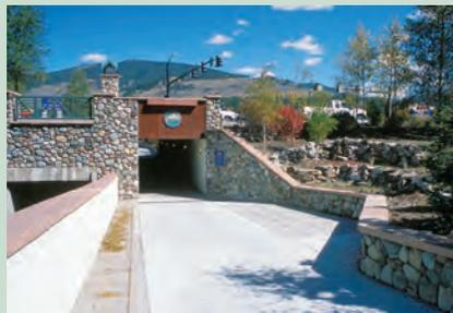
**Ornate.** Both of these tunnels are appealing visual features of the trail, rather than a distraction. In the left photo, the box is wide and provides a shoulder and drainage all the way through the tunnel. In the right photo, the ornate character of the box culvert makes it more of a gateway than an impediment to travel. The hardscape around the entrance is also a visual cue for bicyclists and in-line skaters to slow down.
