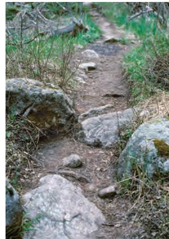
*Even small rocks and/or trees can create a crested squeeze that constrains the tread. Although this is a hiking and horse trail, this approach is appropriate for any trail use.*
