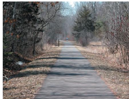
(Left) Proximity close to a road is not ideal but not uncommon when trails are retrofitted. In this case, drainage still works well even though road runoff can run across the trail. With proper grading away from the trail, runoff has little chance to pond or get under the trail surface.
