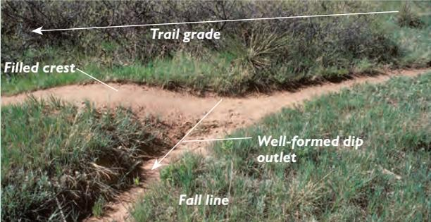
**Excellent filled crest.** Although the crest is small, it's adequate for this hiking-only trail with a stable, well compacted tread.
