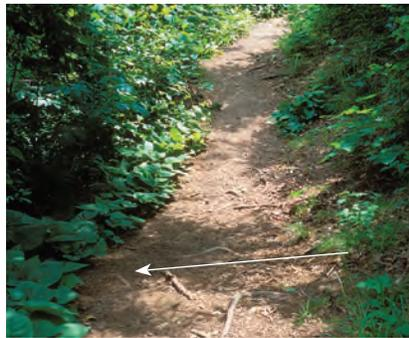
**Correct drainage crossing.** Most drainages crossed are very small and shallow but long enough to not clog.
