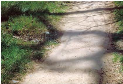
**These crushed stone treads use poured concrete swales to prevent tread erosion by concentrated surface flows.** Both trails are accessible. At left, loose stone particles have collected in the dip, partly clogging it and possibly forming a slipping hazard. At right, the concrete dip is barely visible – crushed stone from the tread itself was used as concrete aggregate and exposed during curing. As a result, concrete color and texture exactly matches the tread.
