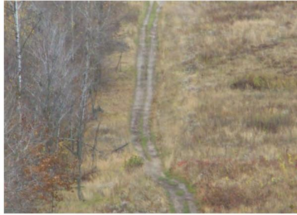
**This rolling grade trail is both fun and sustainable,** in spite of its heavy use. Notice how the dips and crests help manage stormwater and prevent erosion.
