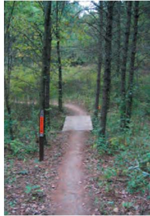
**Anchored bridge** helps ensure that riders will not create a bypass through a drainage, which is ultimately unsustainable.
