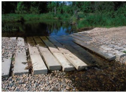
**Water flow undermined small diameter aggregate under some of the planks.** Larger diameter cobbles are needed as a foundation in channels with higher flow speeds.
