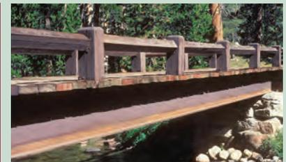
**Thickened edges.** The edges of walls and decks have a stronger and more anchored feel when they are thicker than the rest of the structure. Thickened edges also often create interesting shadow lines.
