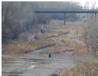
**Trail “freeway”** located in a major greenway in Minneapolis, the Cedar Lake Trail is designed for heavy use. It features a separate two-way trail for walkers and joggers (far left) and two separate one-way trails for bicycles and in-line skaters. The walking trail is 8 feet wide with a 10-foot width used for each of the bicycle trails. This combination has proven exceedingly successful in this setting, but may be more than necessary for most applications outside heavily populated areas.
