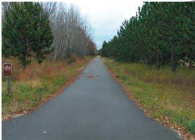
It is common not to provide striping on trails where use levels and hazards are minimal and sightlines adequate. Nonetheless, trail users are responsible to stay in their lane when approaching opposing traffic.
