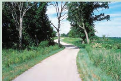
**Relaxed curves.** When there is adequate space in a trail corridor, curves can be laid out to meet or exceed desirable standards and still fit well into the surrounding landscape. In this case, the curvilinear nature of the trail adds considerably to its character.
