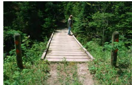
On this ATV trail, bollards are used to make sure that riders are aligned to cross this low bridge. The bollards also help protect the bridge abutment.
