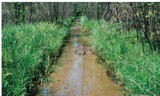
**Wet and level.** This former railroad grade sank in a nearly level area, making it impossible to adequately drain the trail without elevating much of the tread or lowering the local water table. Avoid wet and level, or even nearly level, areas.
