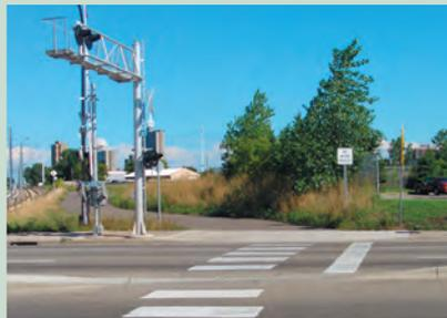
**This midblock crossing has a raised median with a cut through.** This allows trail users to proceed without any ramps or grade changes, so they can focus on the traffic and other trail users.
