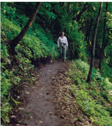
**Ideal, but rare.** This new out-sloped tread has an ideal combination of steep sideslope, stable and cohesive tread material, narrow tread, and low displacement use (hiking). Even out-slope – usually the most difficult tread shape to sustain – is easier to sustain here because of the tread material and use.
