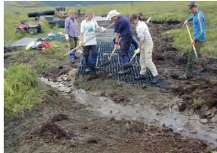
**Hidden paneled drainage crossing.** Ballasted with soil, panels can almost disappear. The top edges of the plastic cells will reappear with trail use when the top layer of soil displaces, but the tread will be laterally unified. Ruts cannot form, displacement and erosion are limited, and plants can potentially grow in the drainage channel and tread for further stabilization.
