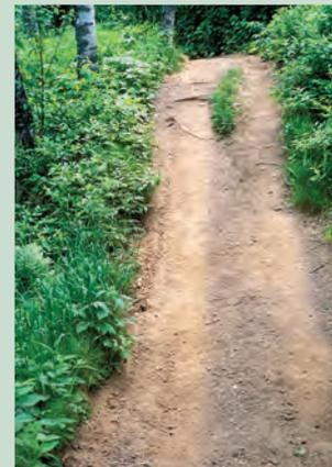
**In-line, climbing.** The trail rolls over a small natural ridge. This short, steep climb is sustainable. Small crests such as this are fun for wheeled uses. (Hiking trail, with ATV tracks from recent trail maintenance)
