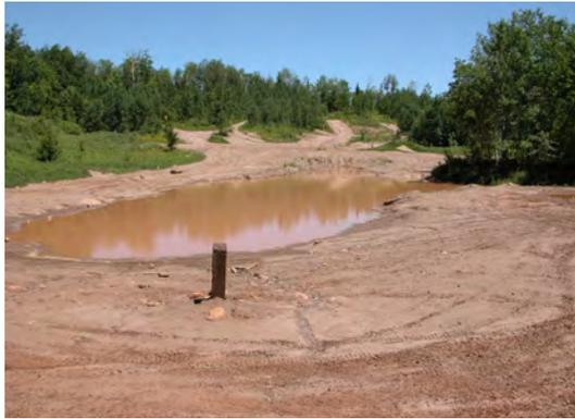
*This water crossing challenge area is purposefully isolated to prevent sediment from getting into larger hydrologic systems. The whole area is less than an acre and is sufficient to meet this limited need.*
