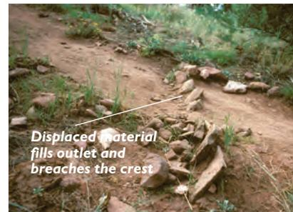
Doomed from the start, this very steep tread grade is close to the fall line. With a very narrow outlet, the waterbar slows water coming down the tread and acts as a settling point for displaced tread material, which breaches the crest.
