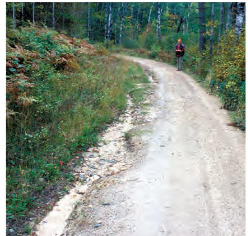
*Years of truck traffic compacted the tread of this long-established on-road trail. The trail erodes, but the eroding channel stays to the softer edge of the active tread. Note that even this gentle grade erodes because it has a large surface area that captures a large amount of rainfall and runoff from the slope at left. Because trail users impart far less compaction force than trucks, trails tend to erode inside their treads rather than beside them.*
