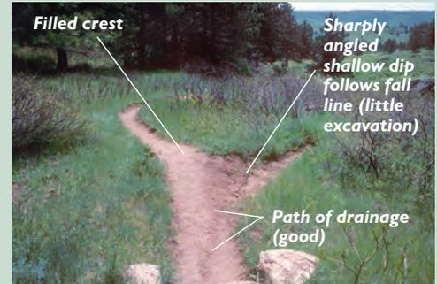
This is an excellent shallow excavated dip that routes water off the trail through a shallow outlet following the fall line. Note the angle of the water path as it enters the dip, where it gradually flows into the dip with a steady grade. The outlet will still occasionally need to be cleaned out.
