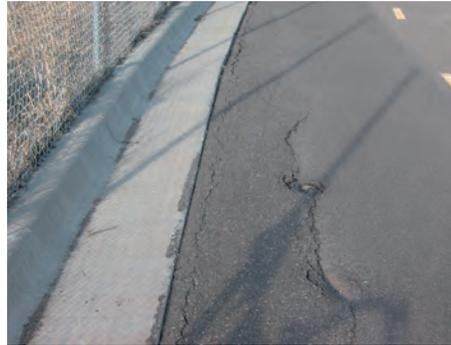
(Left) Where shoulders are too narrow and adjoining sideslopes are steep, edge stability can become a problem. This asphalt patch is only a temporary solution.
