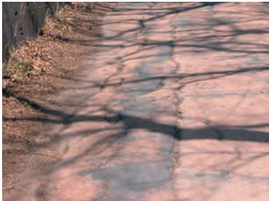
*This trail is simply so old and cracked that an overlay or total reconstruction are the only practical approaches to improving it.*
