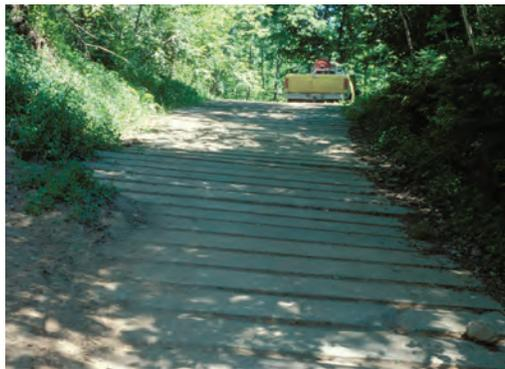
**Displacement is best limited through good design.** Where that is not possible, the tread must be adequately hardened to remain sustainable, as at a stop sign where compacted aggregate can be used in the start/stop zone (left).
