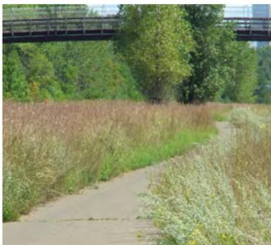
Even prairie grasses can be a significant impediment to travel along a trail. The extensive encroachment along this trail effectively narrows it from 10 feet down to 8 feet and is annoying to many bicyclists. Simply mowing a 2-foot strip on each side would vastly improve this situation. Encroaching vegetation also can shorten the life of a trail by getting under the pavement edges.
