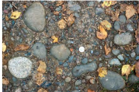
**Firming.** This is done by compressing stony material into the top layer of native soil rather than modifying the entire tread. Firming may sometimes be sufficient for lightweight, low-displacement uses.
