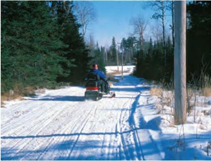
*This is a common example of a comfortable clearance zone adjacent to a groomed and tracked trail. The clearance zone is especially important where trees and brush are present on downhills. Note that by limiting the clearance zone, trail "creep" can be controlled, as can cross-country travel.*
