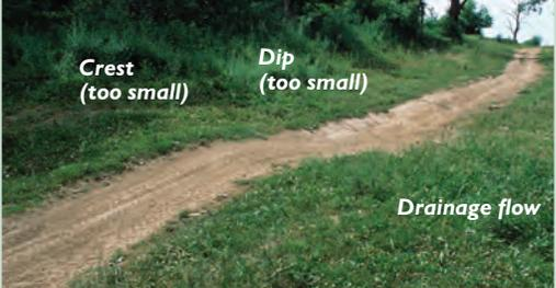
**Partial implementation.** This filled crest is working for now, partly due to very stable tread soil. The crest, however, has little effective volume and the dip is very shallow. In sandy soil, displacement would quickly wear the crest down and sediment would likely clog the dip.
