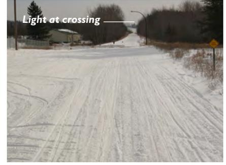
Along with proper signage, a light is added at this trail crossing to improve safety. The flatness and straightness of this trail conversion reduced the visual cues associated with identifying this intersection, warranting the addition of the light.
