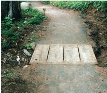
*This timber culvert is simultaneously an anchor, edge, and gateway.*
