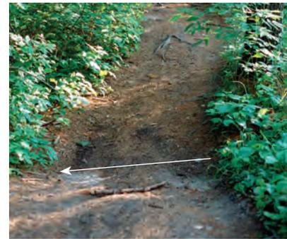
**Correct drainage crossing.** The tread directly crosses a small yet defined runoff channel (the light-colored soil in the immediate foreground). Well-drained soil prevents muddiness on this ATV trail.
