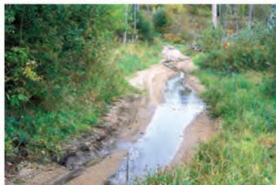
**Incorrect rolling grade drainage crossing.** This trail is intercepting and diverting water from a site drainage crossing behind the photographer, sending it down the tread. If the tread had a rolling grade on the slope at left, this diversion could be prevented.
