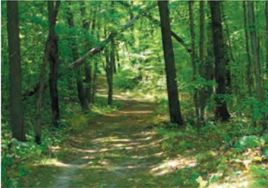
**Limited trail corridor.** The corridor for this hiking trail with compacted soil and vegetated tread is only a few feet outside the trail clearance zone since there is very limited likelihood of erosion or major concentrations of stormwater.
