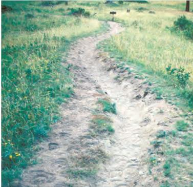
**Horse tread.** Horses flip their hooves as they walk, displacing soil a short distance in all directions. In loose soil, displacement forms distinct berms on each side of the trail. In firmer soils, horse trails can be firmly compacted (desirable).
