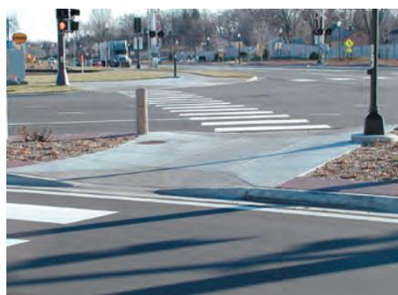
(Right) This landing area is in between the main road and an access ramp to a freeway. Although it is large enough to accommodate a few trail users, the narrow curb forces users to the center of the ramp just when everyone is grouped-up at a constricted point. If the ramp were as wide as the trail, people headed in either direction could stack up beside each with little interference.
