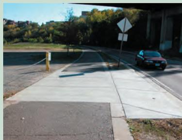
**The use of concrete can help remind trail users to look both ways at a driveway crossing.** The consistent grade is also a positive aspect of this crossing.
