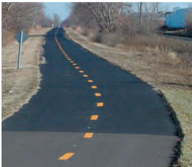
In contrast, this trail has been properly designed with a heavier cross-section on a stable base. It is reasonable to expect 15 years of design life from this trail.
