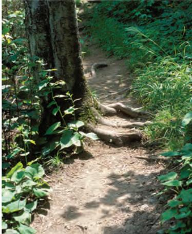
*This tree anchor extends partway into the tread; its exposed roots are part of the tread crest.*
