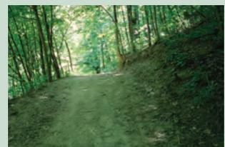
**Shoulder.** A vegetated strip on the outside edge is used to create a greater sense of safety and edge stability. The shoulder is lower than the tread and often slopes slightly down toward the outside edge (outsloped). Ditches are optional. Shoulders are often used on trails formed on railroad grades and roadbeds.
