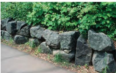
This dry-laid stone retaining wall anchors a trail segment and adds rustic natural shapes and new colors and textures to this asphalt trail. Vegetation overlapping the stones ties the wall into the site.
