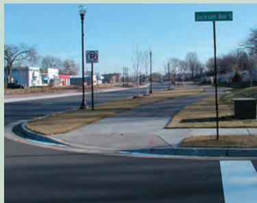
**Standard, appropriately positioned crossing.** This crossing at an intersection works well. The only limiting factor is that the accessible ramp is not as wide as the trail, which can cause problems if bicyclists meet on the ramp and are both forced to the center.
