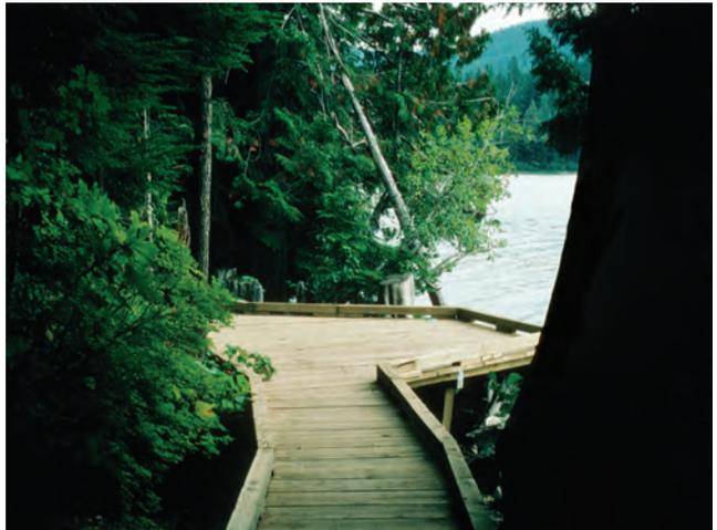
(Above) A high-contrast anchor, such as this viewpoint, is very compelling and attractive to visitors. The deck helps anchor the trail and also uses natural shapes (segmented curves in lumber) to wrap around the large tree at right, which in turn ties the two together into a natural form. The raised, extended deck provides a vista through the trees, while at the same time discouraging visitors from leaving the trail.
