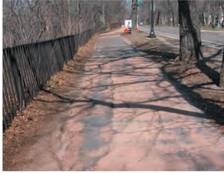
(Left) The longitudinal crack in this trail is a classic example of an unstable or inadequately compacted subgrade. The only real solution is to rebuild it.
