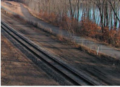
A chainlink fence was used along this trail/rail corridor to provide safe separation between uses.
