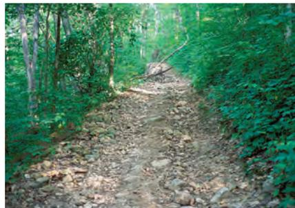
**Rough tread sections formed through use.** Trying to create “rough” sections can be a challenge and cause additional site impacts. It’s best if rough sections are formed through trail use, as long as they remain sustainable).
