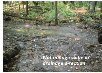
Inadequate dip outlet slope causes standing water in the dip. Even though the dip outlet, foreground, is wide, the outlet slope is not steep enough to adequately drain water from the tread.
