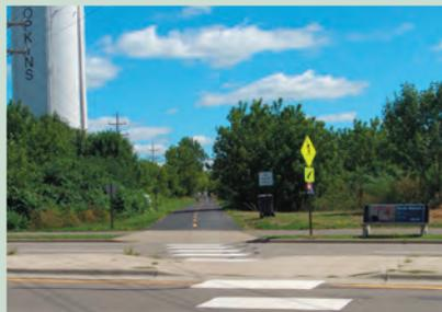
**Raised island with partial ramp cut-through.** Although the island is a good idea, the cut-through is too narrow, which forces opposing trail users to wait in the middle of the road to pass one at a time. This can pose a safety risk when motorized traffic is approaching from both sides.
