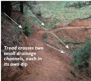
**Suitable technique.** On this steep sideslope, the trail is aligned relatively level and curved around the inside of the drainage to minimize tread erosion and improve safety. Enough of a dip must be provided to keep water in the drainage. In this case, the limited drainage requires only a small dip at each crossing.
