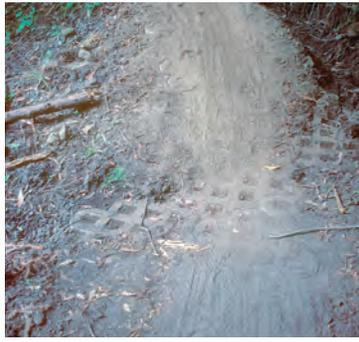
**Interlocking concrete block** (left) was used to harden both the approach and the drainage crossing. While not natural, it effectively controls displacement and erosion. Extensive use of concrete block is recommended only where more natural hardening methods are not feasible. Note that one of the main advantageous of blocks over stones is that they interlock, creating a stronger bond.
