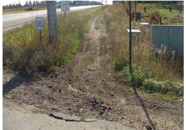
**Problem: Increasingly unsustainable impacts to driveway approaches.** In each of these cases, the loss of stabilizing vegetation and rutting/displacement of soils is exposing the pavement edge and undercutting its structural integrity. Of all the conditions that concern local roadway engineers, this is the one that gets the most immediate attention simply because of the safety concerns and ongoing maintenance costs.
