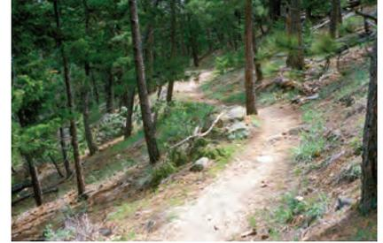
**Wise use of the site.** Trees and rocks on this slope anchor a gentle rolling grade. The many twists and turns through the trees with slight roller-coaster ups and downs makes the trail engaging. The hiking trail uses outslope for some drainage and tread dips where an edge protection buffer has formed.
