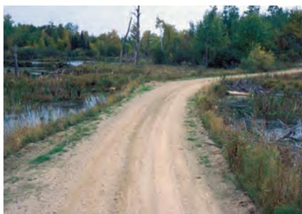
**Wider tread may be needed.** On easier trails, treads can be up to twice the normal width in places such as blind curves or where trails come together at odd angles (left).
