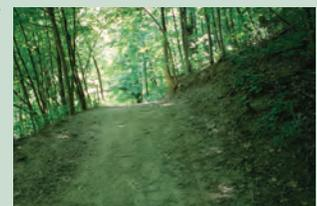
**Shoulder.** A vegetated strip on the outside edge is used to create a greater sense of safety and edge stability. The shoulder is lower than the tread and often slopes slightly down toward the outside edge (outsloped). Ditches are optional. Shoulders are often used on trails formed on railroad grades and roadbeds.
