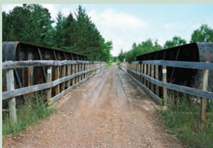
**Bridge designs to be cautious about.** In the left photo, the bridge is only 8 feet wide, which is less than the adjoining trails. This can cause conflicts if those using the trail do not go single file across the bridge. In the right photo, the planking runs in the direction of the trail. If used for ATVs or horses, this poses few problems. But bicycle tires can catch on the edges and throw the rider off balance.
