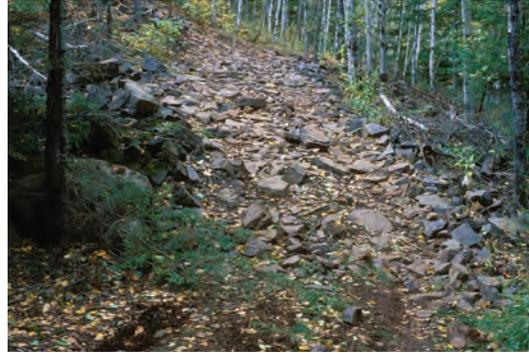
**Hardening material found near the site.** In many cases, well-graded pit run gravels can be used for tread hardening to create a stable trail at reasonable cost (left). For some uses, hardening also serves as a trail challenge, as is the case with this OHV trail in an OHV recreation site (right). Both of these will likely prove to be very stable over an extended period of time.
