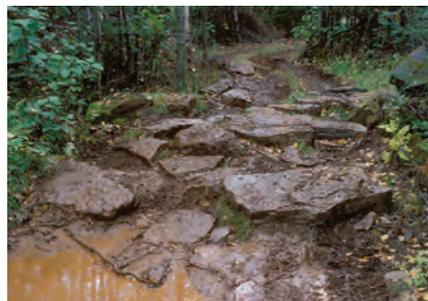
**Native or imported rocks provide many challenges.** For stability and anchoring, the larger the obstacle, the better. Rocks and boulders can be used to require skillful negotiation with narrow clearance and create rough tread to cause vehicle articulation (left).
