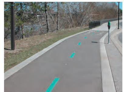
In some systems, a green center line is used in lieu of yellow as an identifier of a system of trails. If this approach is taken, maintain consistency to avoid confusion.
