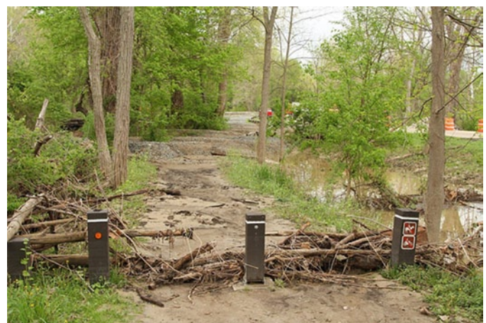
Erosion damage to stone dust trail.
