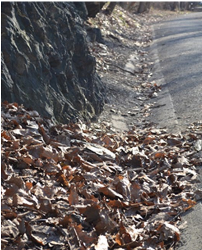
Drainage swale in need of cleaning.
