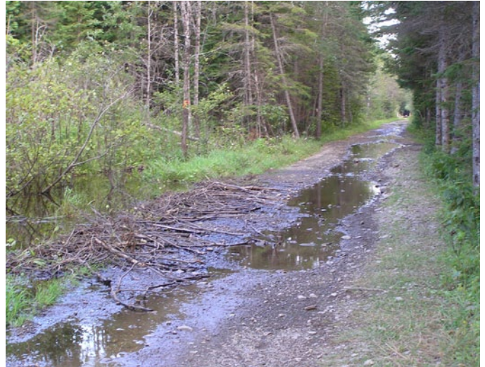
Beaver caused erosion damage, Ashuelot Rail-Trail, NH.
