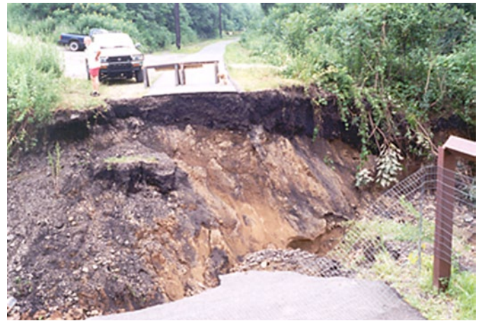
Culvert failure, Allegheny River Trail, PA.
