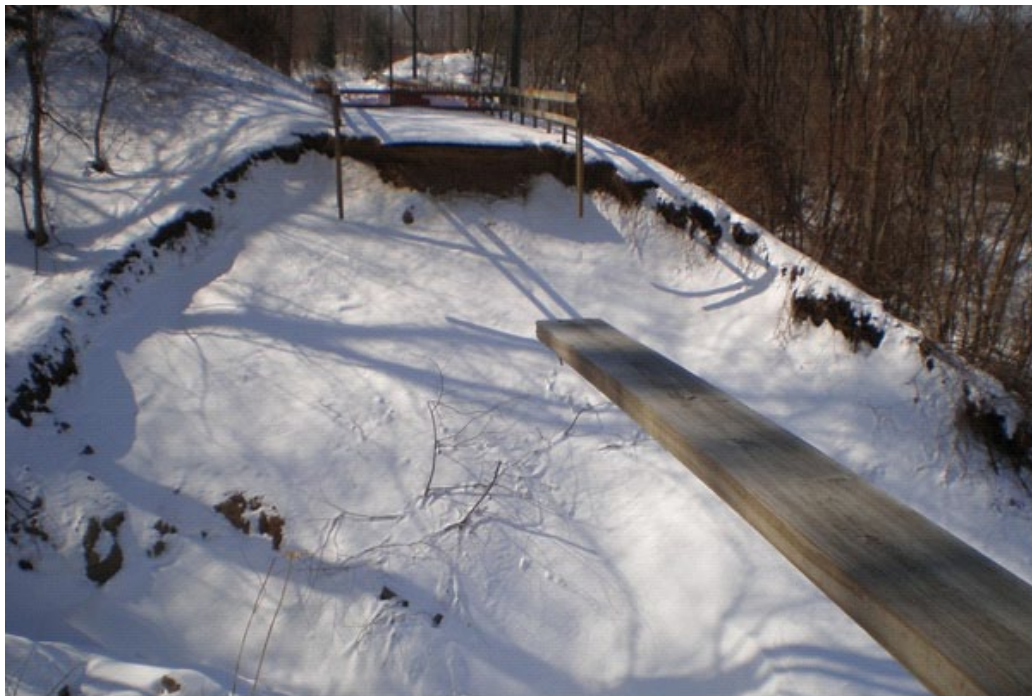
Culvert failure, Manhan Rail Trails, MA.
