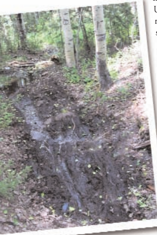
Water on trail promotes rutting and widening. (Brain Head, UT)
