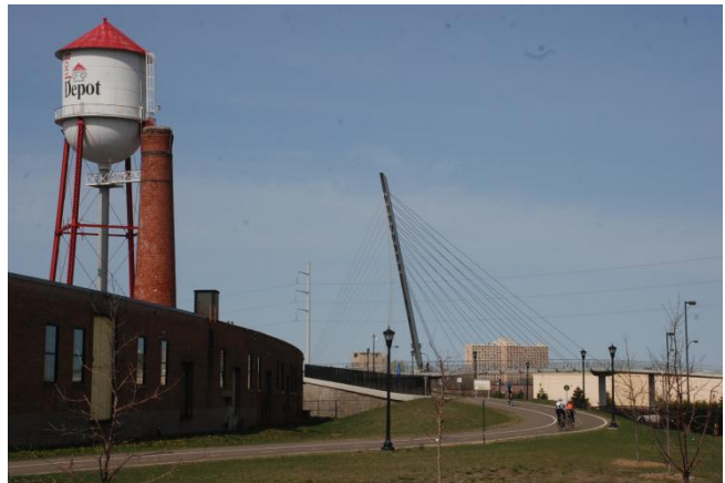
Photo 3 - The Martin Sabo Bridge, constructed in 2007, connects Phases II and III of the Midtown Greenway over Hiawatha Avenue and the Hiawatha LRT line. (photo by the author, 2010)
