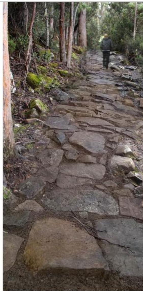
**Proposed:** Water pipe to be relocated away from the track. Harden steep track section with informal dolerite paving.
