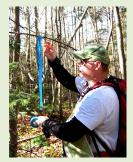
New trail will be marked either at the centerline, inside edge or critical edge. A trail may also be broken down into sections marked with stakes marked with standard civil engineering notation (1+00, etc.) that will correspond with the project notes/construction notes. Flagging can also mark special features for a Crew Leader to be aware of such as hazards, structure locations or obstacles for removal.
