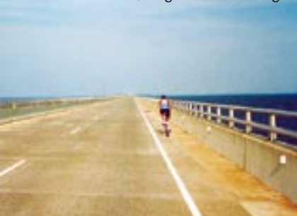
4. Croatan Sound/Virginia Dare bridge
