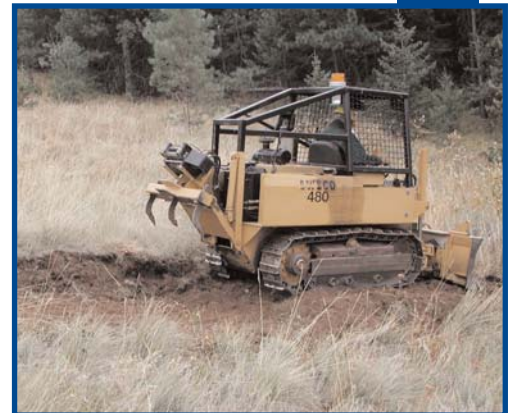
Mechanically constructed rolling dips or undulating trail grades provide water control and reduce
