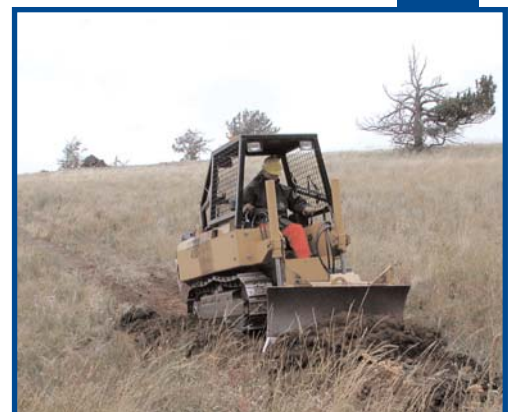
Mechanically constructed rolling dips or undulating trail grades provide water control and reduce
