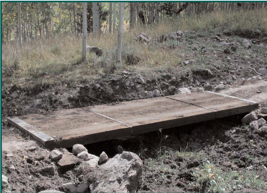
Harden or bridge stream crossings where appropriate to reduce sediment delivery.
