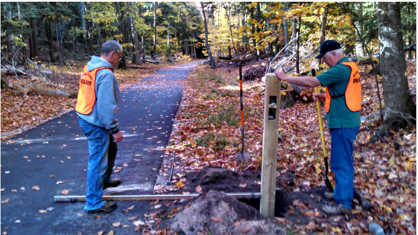
Figure 10-2: Installation of a pedestrian counter at Sleeping Bear Dunes National Lakeshore. (Source: NPS)
