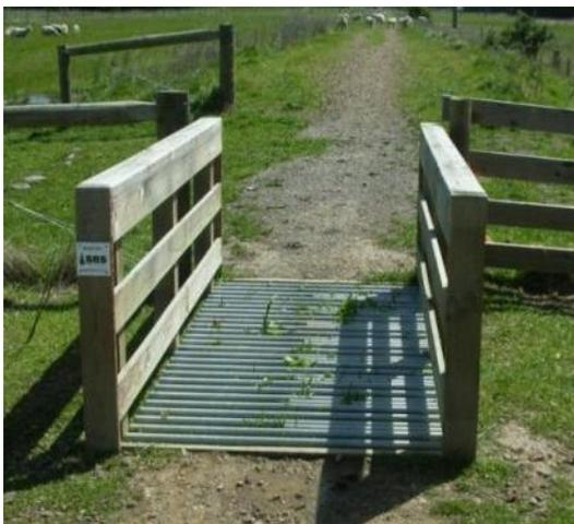
Figure 55: Cattle stop placed on straight alignment of track
