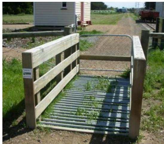
Figure 56: Gate added – a poor solution for cyclists
