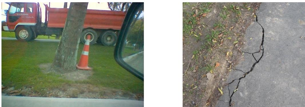
Figure 25: Heavy truck causing edge break on new pathway during construction
