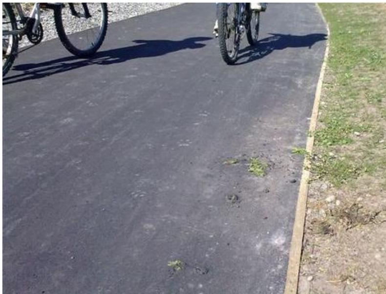
**Figure 85: Vegetation growing through new asphaltic concrete path; good construction specifications and contract supervision are required**
