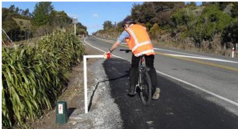
**Figure 38: Push button activated warning sign at vertical crest, SH 60 near Nelson (photo: NZTA)**
