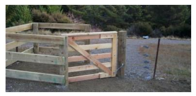
Figure 60: Kissing gate: Hawea Track; can be difficult for tandems and bikes with trailers
