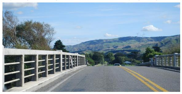
Figure 48: Many railway overbridges have inadequate shoulder width and may require clip-on bridges on each side for cyclist safety (photo: Jonathan Kennett)
