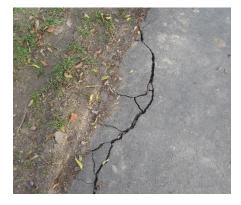
Figure 25: Heavy truck causing edge break on new pathway during construction
