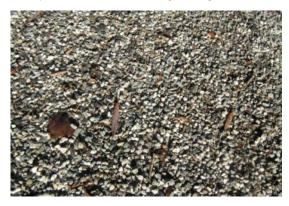
Figure 24: Chip seal path in Queenstown
