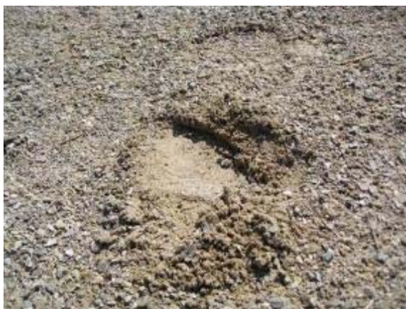
Photo 138 Quarter Inch Minus Limestone trail segment would only firm up after extended periods of no moisture. March 17, 2009.
