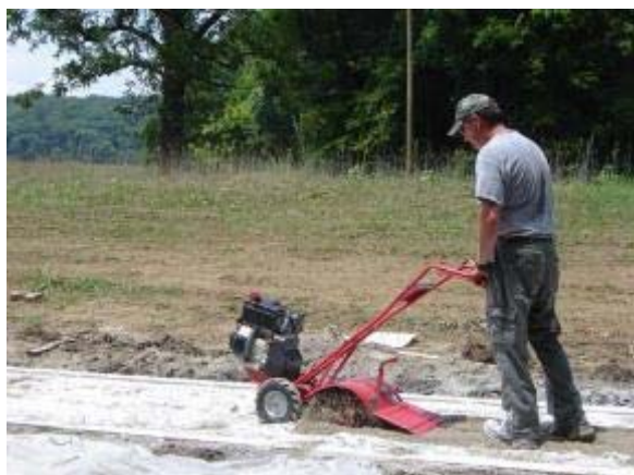
Photo 30 Soiltac Powder Mix-In is tilled into the 2 inch base of native soil. June 27, 2007.
