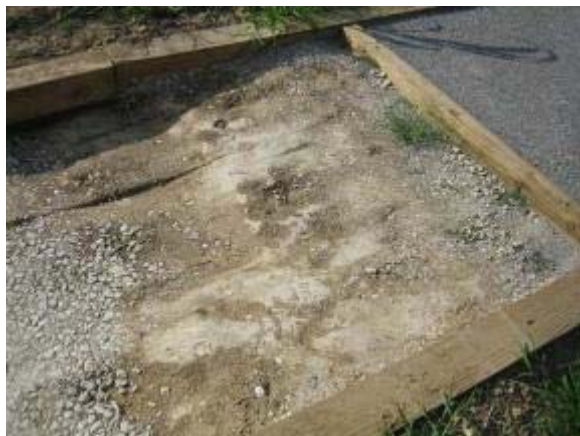
Photo 133 Quarter Inch Minus Limestone was installed in two rolled and compacted 3 inch lifts. August 9, 2007.
