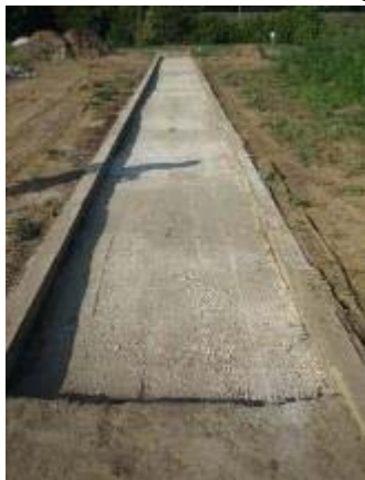
Photo 139 Three Quarter Inch Minus Base and Quarter Inch Minus Top Limestone trail segment is composed of 4 inch base; and a 2 inch top-dressing. August 9, 2007.
