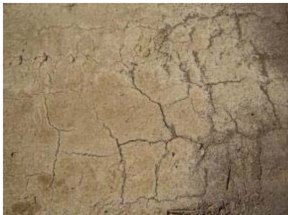
Photo 112 Polypavement trail segment shows cracking. July 6, 2007.
