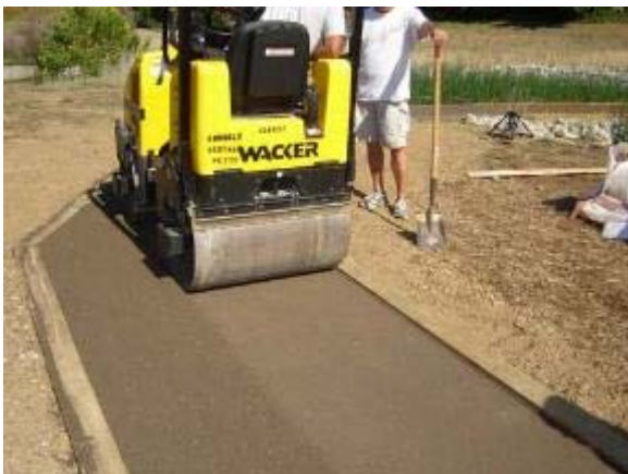
Photo 94 StaLok surface is compacted. June 21, 2007.
