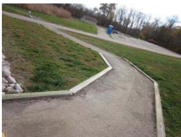
Photo 106 StaLok trail segment had some pooling of water at lower points of the surface. November 2, 2011.
