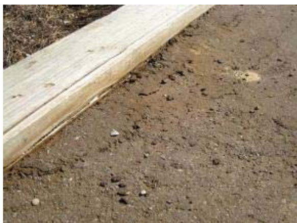
Photo 98 StaLok trail surface had a pattern of wear and repairing itself. March 13, 2008.
