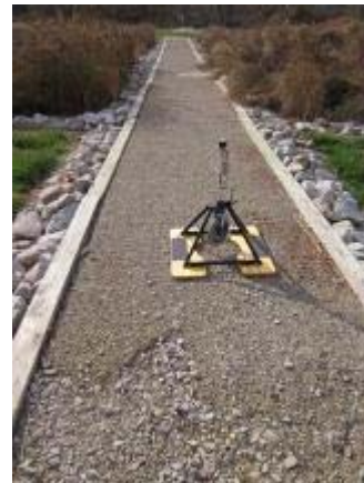
Photo 16 Klingstone at beginning of trail segment has started to wash out. November 22, 2011.
