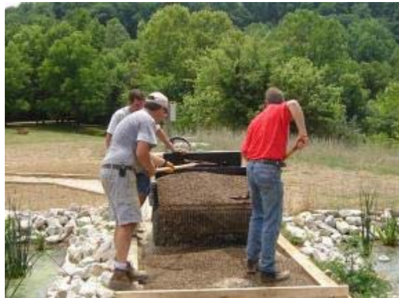
Photo 4 Klingstone top dress \frac{3}{4} inch washed pea gravel is prepared. June 16, 2007.
