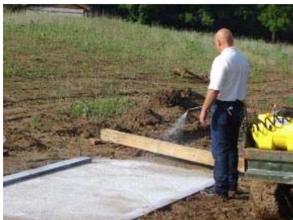
Photo 43 Soiltac Liquid Topical is applied to a base of 2 inch native soil, mixed with water and sprayed onto 4 inches of \frac{1}{4} minus compacted limestone aggregate. June 27, 2007.
