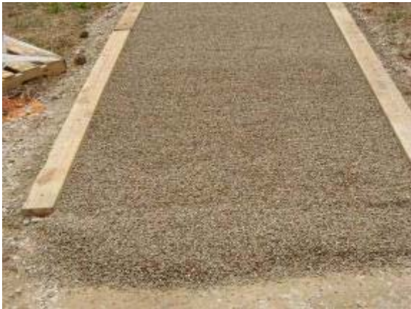
Photo 3 Klingstone top dress preparation of \frac{3}{4} inch washed pea gravel (round river rock). June 16, 2007.
