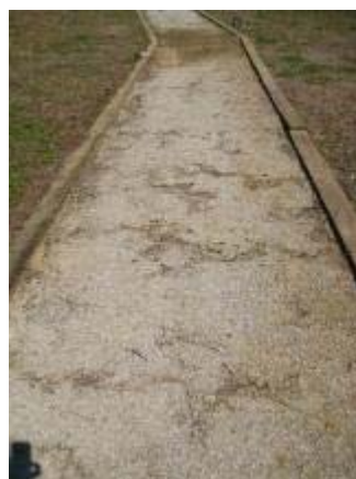
Photo 66 Soiltac Liquid Mix-In almost two years after installation. March 17, 2009.
