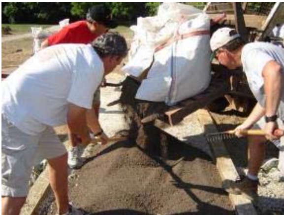
Photo 92 StaLok is applied at a 2 inch depth on top of the base. June 21, 2007.
