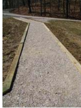
Photo 129 Three Quarter Inch Minus Limestone trail segment where water pooled after rain. March 13, 2008.
