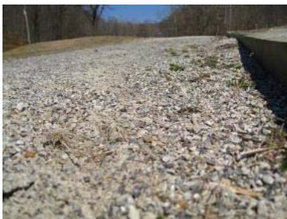
Photo 86 Stabilizer trail segment shows deterioration from runoff along timber edging. March 17, 2009.
