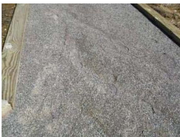
Photo 80 Stabilizer trail segment has runoff from heavy rainfall. March 13, 2008.
