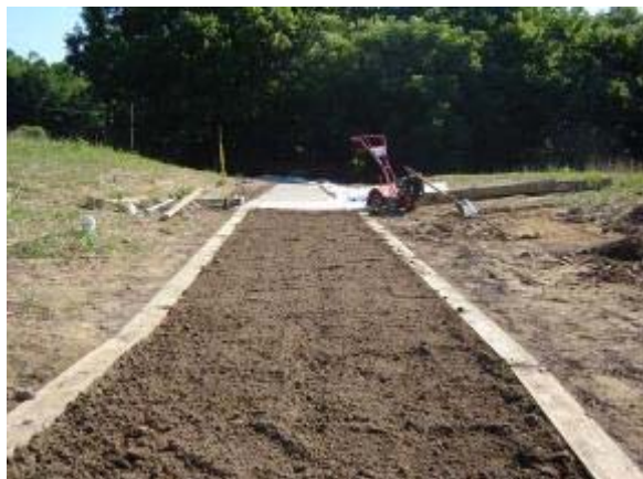
Photo 108 Polypavement is applied to a base of compacted native soils and mixed into an additional 2 inches of tilled soil. July 3, 2007.
