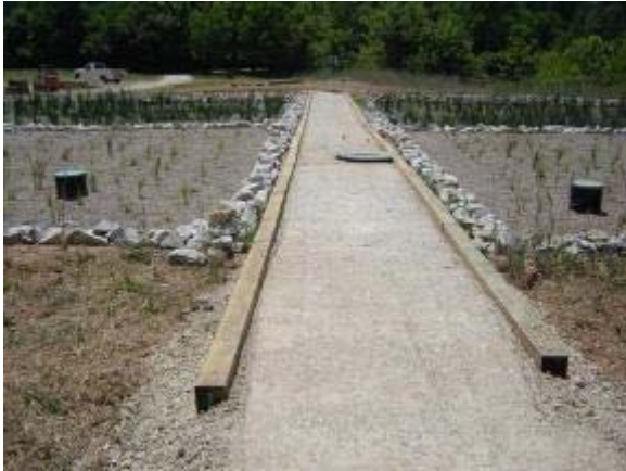
Photo 1 Klingstone base preparation of \frac{3}{4} inch minus limestone and dust. June 13, 2007.
