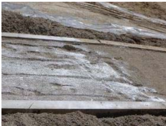
Photo 29 Soiltac Powder Mix-In is applied to a base of 2 inches of native soil. June 27, 2007.
