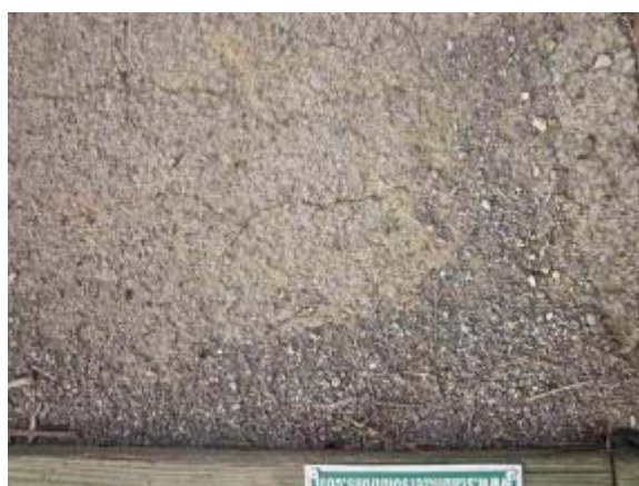
Photo 105 StaLok trail segment shows cracking next to timber edging. November 2, 2011.
