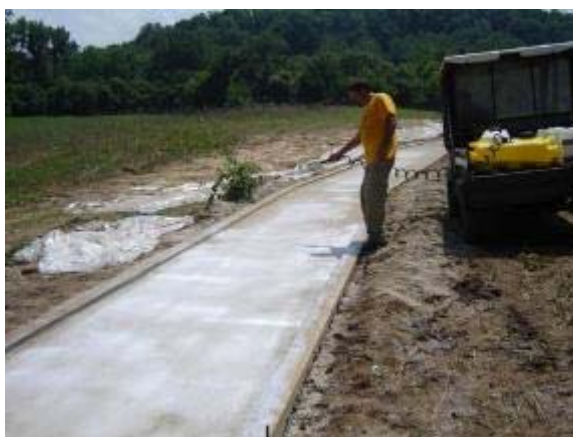
Photo 62 Soiltac Liquid Mix-In trail segment is sprayed to seal with a penetration of 4 inches. June 27, 2007.
