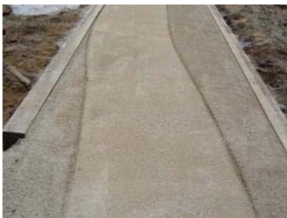
Photo 33 Soiltac Powder Mix-In is smoothed and compacted. June 27, 2007.
