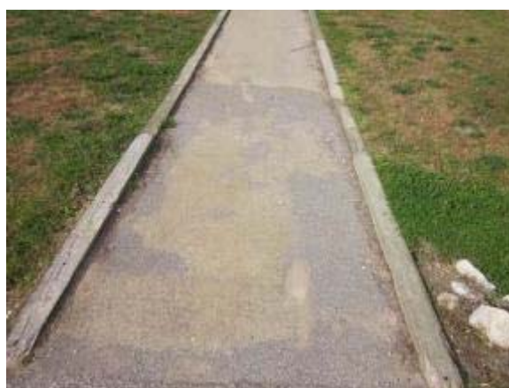
Photo 107 StaLok trail segment with pooling of water. November 2, 2011.
