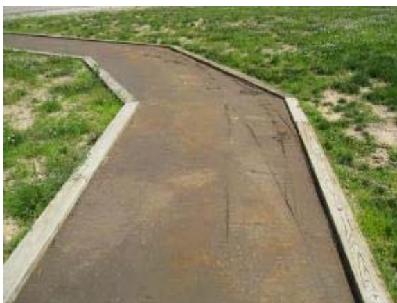
Photo 101 StaLok trail segment with wheelchair marks would repair itself. June 12, 2008.
