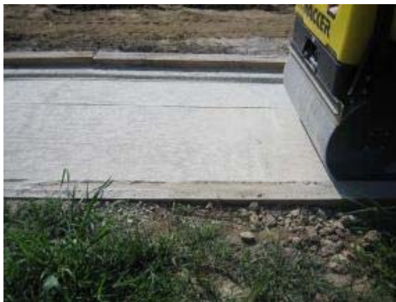
Photo 134 Quarter Inch Minus Limestone trail segment as second lift is rolled and compacted. August 9, 2007.
