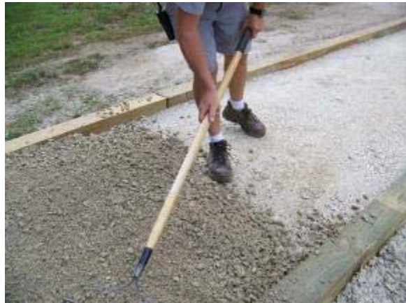
Photo 125 Three Quarter Inch Minus Limestone trail segment has second lift installed. August 3, 2007.
