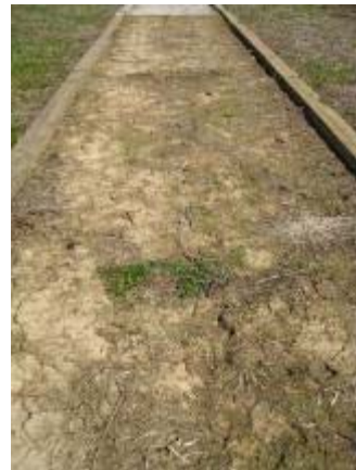
Photo 119 Polypavement trail segment almost two years after installation shows top layer of stabilizer and remaining surface returned to its natural soil base. March 17, 2009.
