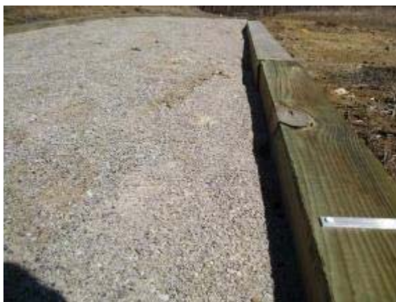
Photo 136 Quarter Inch Minus Limestone trail segment was loose under foot after heavy rainfall. March 13, 2008.
