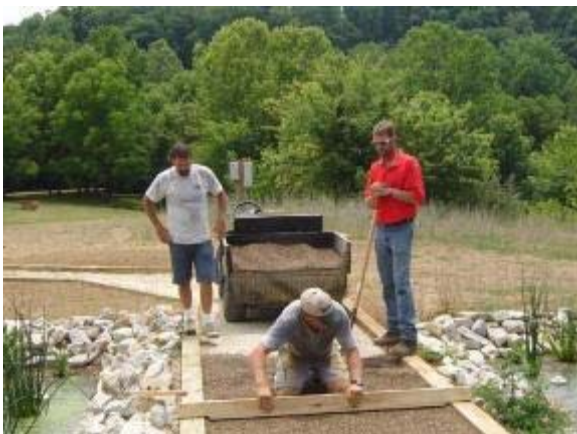
Photo 5 Klingstone top dress \frac{3}{4} inch washed pea gravel is leveled. June 16, 2007.
