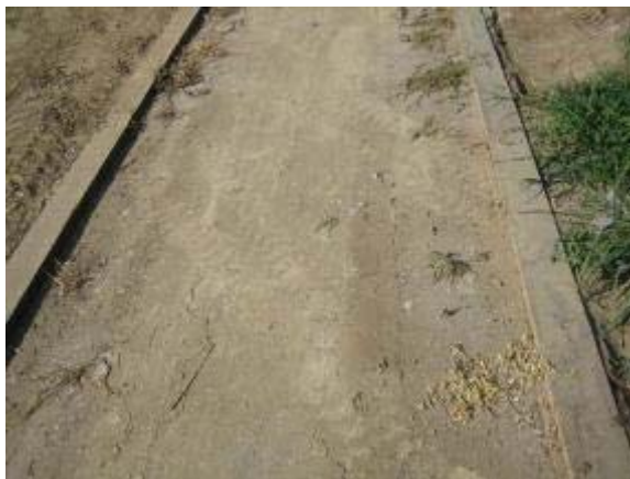
Photo 113 Polypavement trail segment after heavy rains remained cracked. August 9, 2007.
