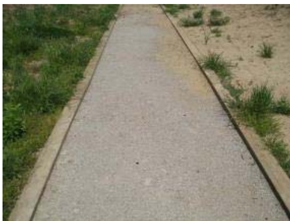
Photo 48 Soiltac Liquid Topical trail segment remained soft where water had pooled. May 6, 2008.
