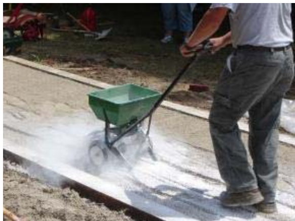
Photo 28 Soiltac Powder Mix-In is applied to a base of 2 inches of native soil. June 27, 2007
