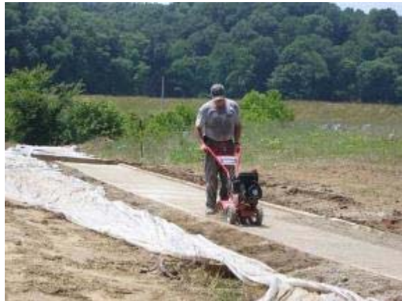
Photo 58 Soiltac Liquid Mix-In surface is tilled. June 27, 2007.
