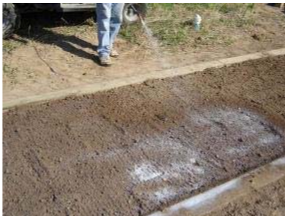
Photo 109 Polypavement is applied to a base of compacted native soils and mixed into an additional 2 inches of tilled soil. July 3, 2007.
