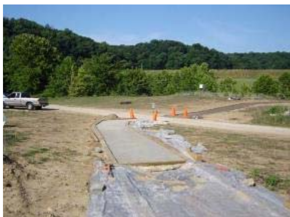
Photo 75 Stabilizer trail segment installation. July 3, 2007.
