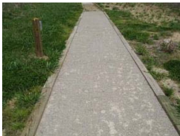
Photo 142 Three Quarter Inch Minus Base and Quarter Inch Minus Top Limestone trail segment firmed back up more quickly than the ¾ inch surface. May 6, 2008.
