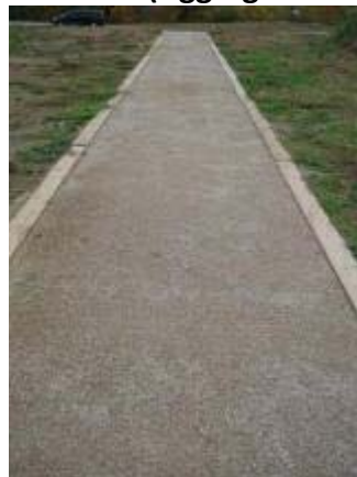
Photo 140 Three Quarter Inch Minus Base and Quarter Inch Minus Top Limestone trail segment maintained itself in dry temperatures. October 19, 2007.
