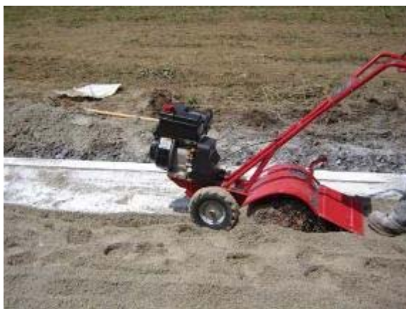
Photo 31 Soiltac Powder Mix-In has a penetration depth of 4 inches. June 27, 2007.
