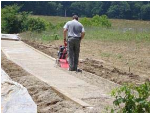
Photo 57 Soiltac Liquid Mix-In is then tilled into 4 inches of \frac{1}{4} inch minus loose limestone aggregate. June 27, 2007.
