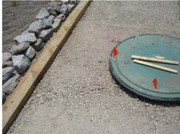
Photo 2 Klingstone base preparation of \frac{3}{4} inch minus limestone and dust. June 13, 2007.
