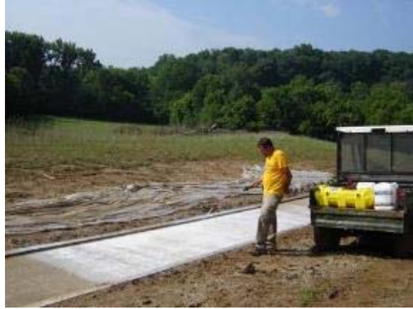
Photo 19 Soiltac Powder Topical is applied to a base of 2 inches of native soil and 4 inches of \frac{1}{4} inch minus compacted limestone aggregate. June 27, 2007.
