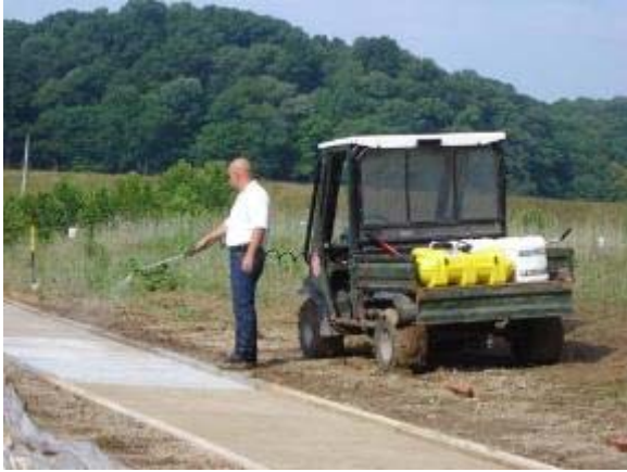
Photo 18 Soiltac Powder Topical is applied to a base of 2 inches of native soil and 4 inches of \frac{1}{4} inch minus compacted limestone aggregate. June 27, 2007.
