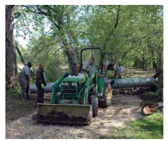
FIGURE 22. Install a culvert pipe which can handle high water and is flush with the stream bottom with rocks around the upstream end to reduce erosion. *Photo by Doug Rowley, National Park Service.*
