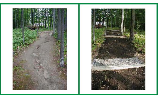
FIGURE 17. Trail before and after waterbars were installed to divert water off the tread. Waterbars should be installed only as a last resort. *Photo courtesy of Maine Department of Environmental Protection, Bureau of Land and Water Quality.*
