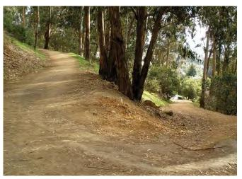
FIGURE 18. Switchbacks help the user traverse a steep slope at a comfortable pace. *Photo by Ken Cheetham.*
