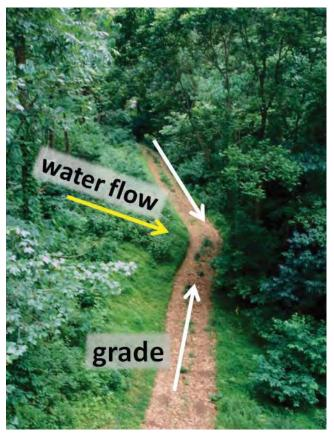
FIGURE 16. A rolling grade uses undulating crests and dips to divert water off the tread. *Photo by John M. Randall, The Nature Conservancy, bugwood.org.*
