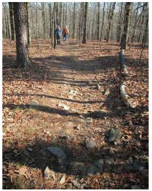
FIGURE 3. This cup-shaped trail forces water down its center and is not sustainable. Rocks, side logs and other debris that funnel water onto the trail should be removed periodically. *Photo by Becky McPeake, UA Division of Agriculture, Cooperative Extension Service.*
