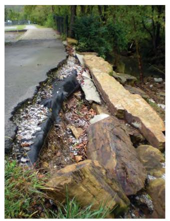
FIGURE 6. This trail was built too close to the stream. Buffers reduce soil erosion, improve water quality and provide habitat for wildlife. *Photo by John Pennington, UA Division of Agriculture, Cooperative Extension Service.*
