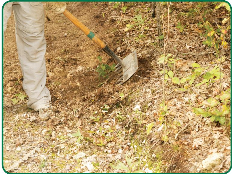
The backslope is cut in from the existing slope down to the tread.
