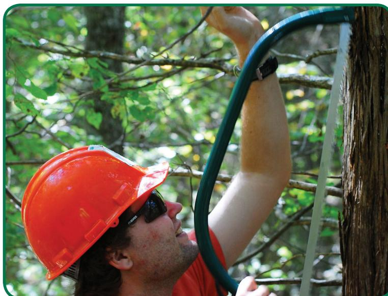
Trimming overhanging limbs is an important part of ongoing corridor maintenance.
