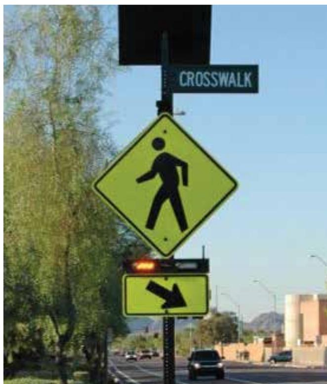
An example of a flashing beacon to alert drivers of the presence of crossing pedestrians | Photo courtesy Institute of Transportation Engineers
