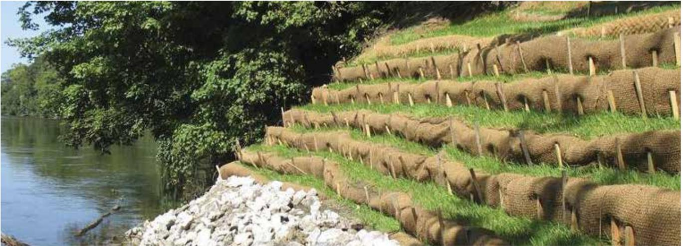
*An example of terracing and slope stabilization | Photo courtesy NBAC*
