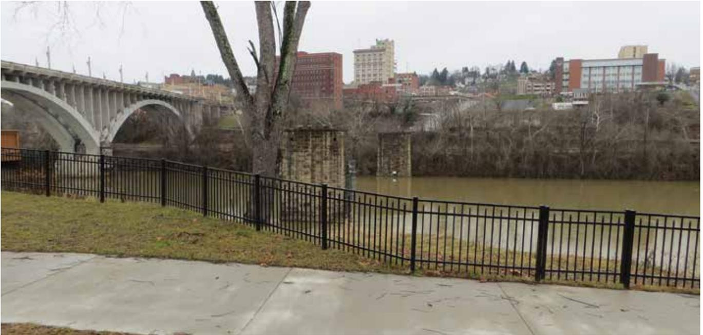
*The Nickel Bridge (or Low Level Bridge) in Fairmont, West Virginia, was removed, but a new bridge can be constructed on the remaining abutments. | Photo courtesy RTC*
