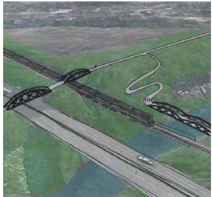
*A rendering of Option 2, including all three new bridges needed to cross US 50, the active CSX line and the West Fork River | Photo courtesy NBAC*
