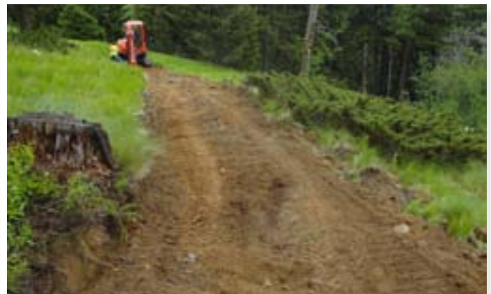
Equipped with a 6-way blade, this excavator is a versatile trail making machine.
