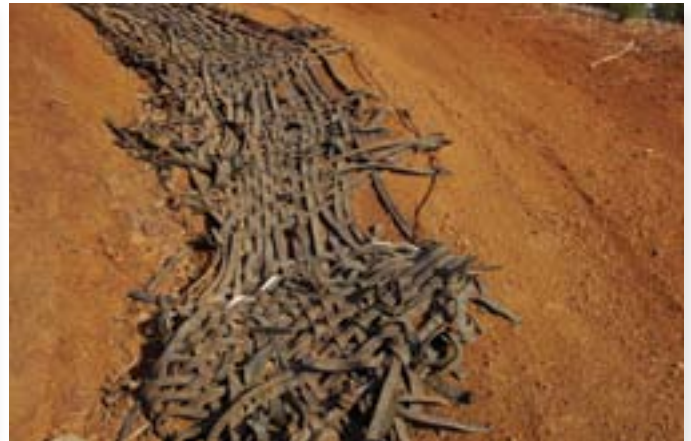
Right and above, once again, the key to success is keeping the material anchored. Once it is allowed to move, it will self-destruct.
