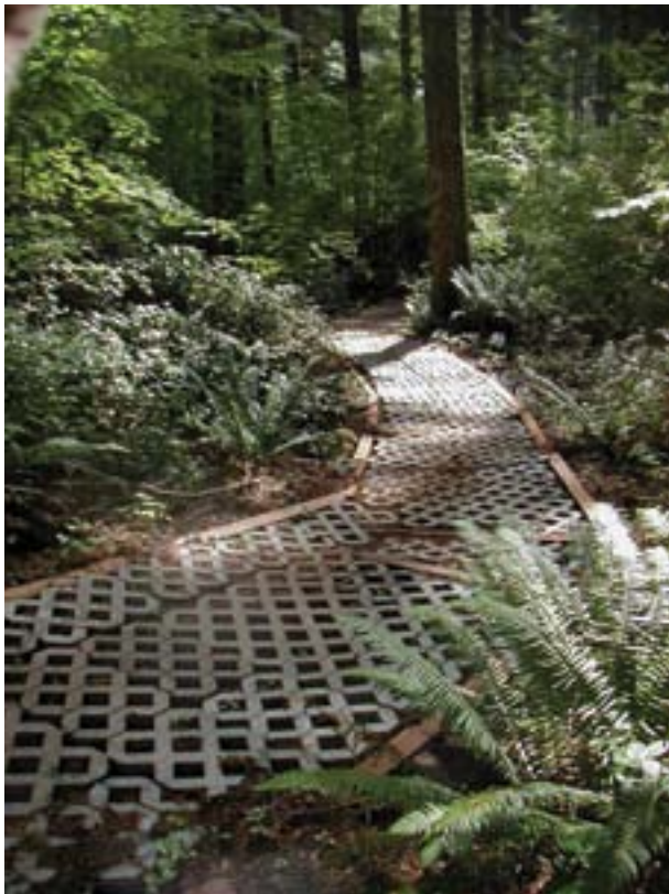
This installation has been framed in which not only resists movement, but provides lateral support and decreases the chance of breakage.
