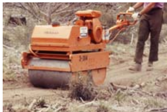
this tandem-drum walk behind vibratory roller is labor-intensive, but it produces a well-compacted product.
