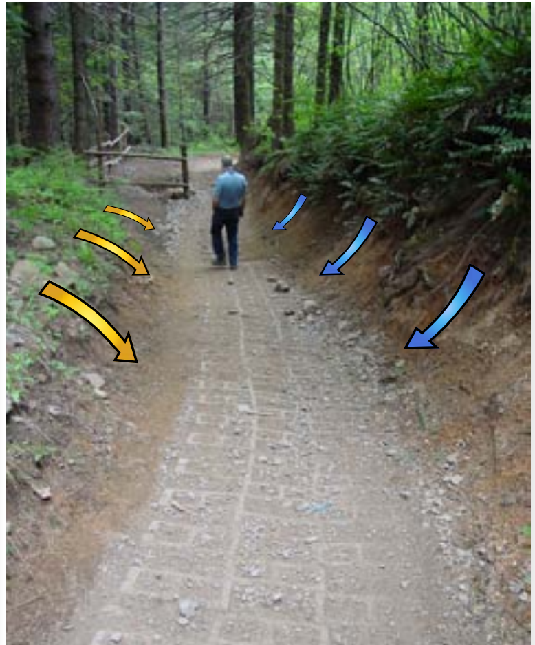
The eroded trench of this site provides natural containment for the blocks. The fill is a densely-graded aggregate that is holding together nicely.
