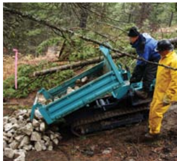
A rock check dam being constructed to control erosion and stabilize a gully created by an old hillclimb.
