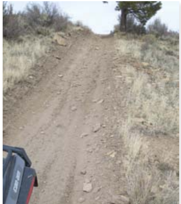
The high rock content on this grade has made it durable. The grade is steep (25%) but short (50'). In spite of a dramatic increase in use, this slope has changed little in 15 years of monitoring.
