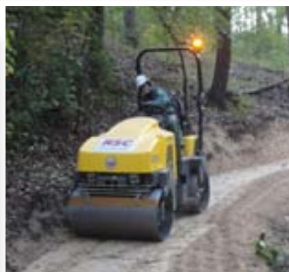
Moist soil will compact better than dry soil, so try to time compaction operations during periods of favorable moisture content.
