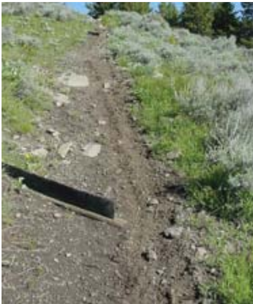
This trail has a long, steep grade, and poor soil type; all ingredients of non-sustainability. Like the rolling dips in roads, these belted waterbars reduce the distance that water runs thereby reducing the size of the tread watersheds. Unfortunately, these won't work. As you can see, riders are already starting to ride around the waterbars and as soon as this happens, ruts will form to channel the water and bypass the waterbars. The result is failure. A bandage fix like this is all too common and it doesn't address the root of the problem: poor trail location.
