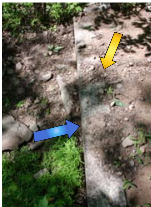
This treated timber waterbar provides a formidable obstacle from below (blue arrow) and being full of sediment, it provides ineffective drainage (yellow arrow). The issue: the tread watershed is too large. Poor soils cannot sustain this grade that is too steep for too long. The solution: relocation.
