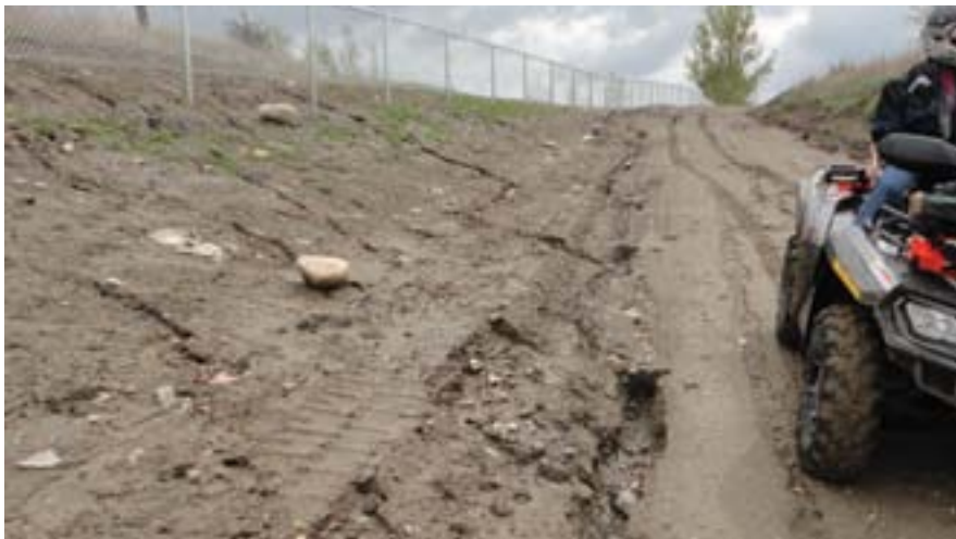
Notice the rills of water draining down the slope and into this trail. Notice also how quickly the rill down the edge of the trail deepens as more water feeds into it and the water velocity increases.
