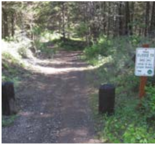
These bollards and gate serve as width restrictons to keep larger vehicles from accessing the trail.
