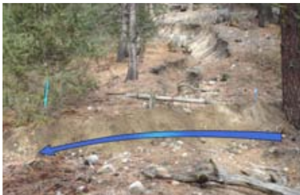
Before rehab efforts could begin on this heavily eroded trail, the source of the water had to be diverted away by ditching it into the natural drainage courses.
