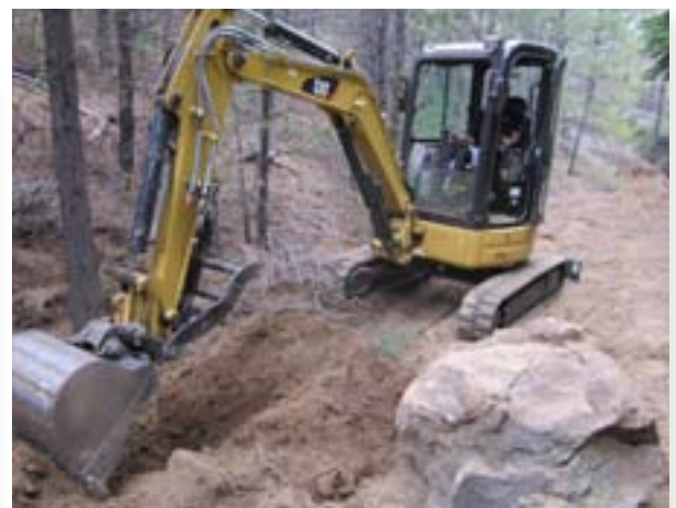
The operator is digging a hole to plant a boulder for a road-to-trail conversion.
