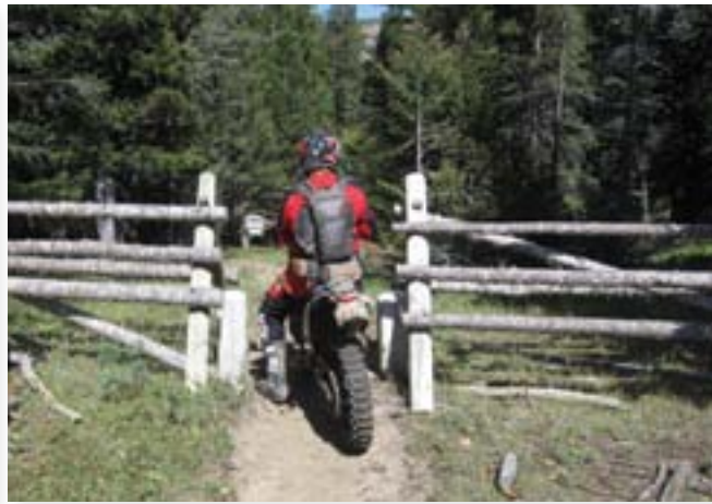
These bollards and gate serve as width restrictons to keep larger vehicles from accessing the trail.
