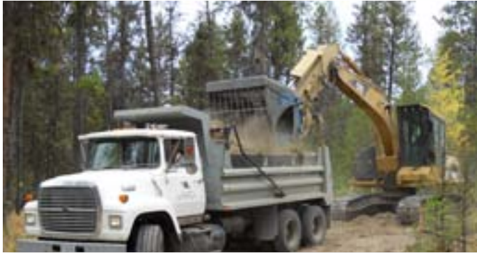
A clamshell bucket is also very handy for plucking trees, stumps, or rocks. This one has a built-in grizzly that allows dirt and smaller rocks to fall through.
