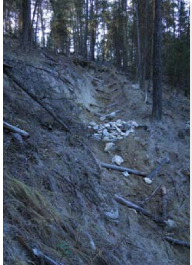
Here, water quality and sedimentation were an issue. Woody debris was placed in a herringbone pattern between rock check dams in a heavily eroded trail leading to a creek that feeds the community water intake.
