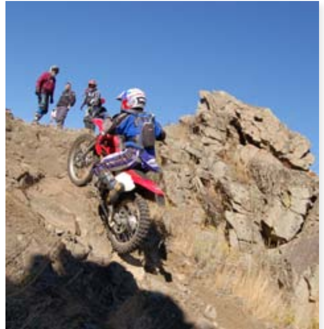
This trail uses a short, but steep climb, to add challenge. The steep grade is stable because the tread is made up of large rocks firmly embedded in the soil.
