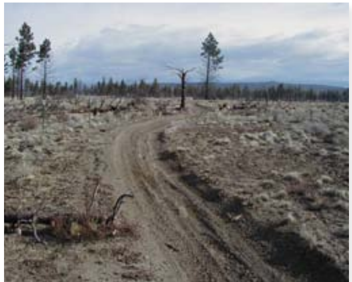
It was a struggle to revegetate this road corridor. Seed was tried first and failed. Next transplanting was done and it failed also. Finally, a wildfire burned it and the next spring, it looked great.
