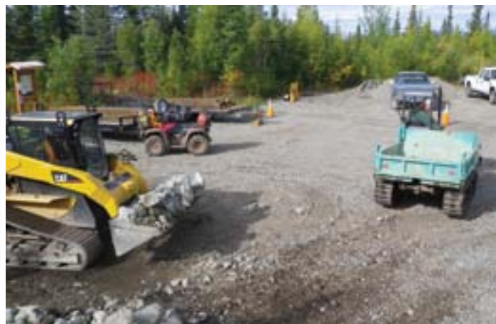
Sometimes sizable areas are needed for staging equipment and materials.
