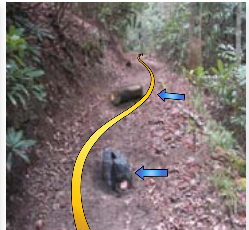
Strategically placing readily available material can produce a significant difference in the horizontal alignment.
