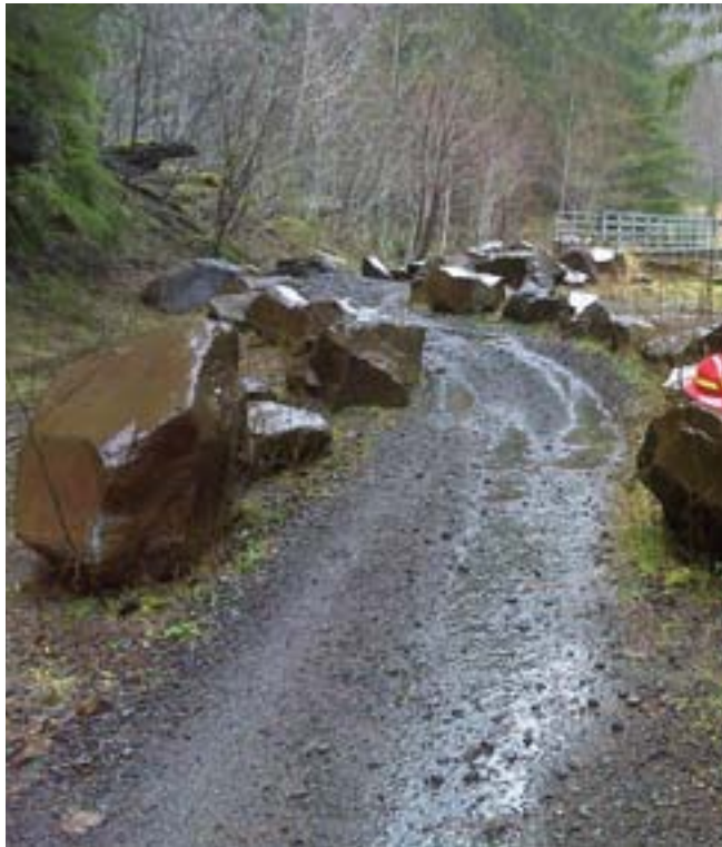
Rocks define a serpentine corridor which slows the riders before approaching the bridge. In this wet environment, this old road corridor will quickly transform into a great trail.
