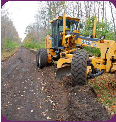
Trail Construction Black Diamond Trail Luzerne County
