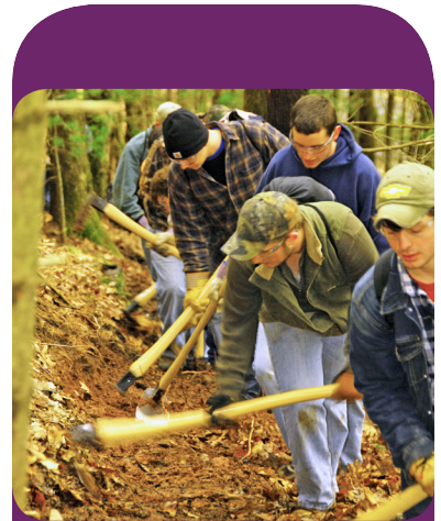
Tread Construction by Hand
