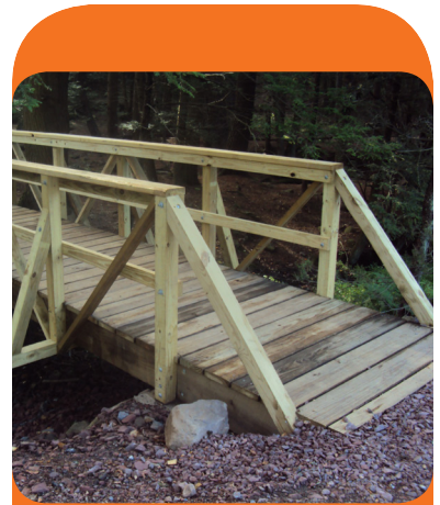
Stringer Bridge Nescopeck State Park Luzerne County
