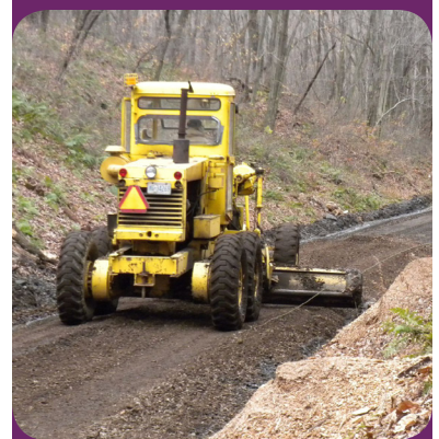
Rail Trail Tread Construction with Road Grader
