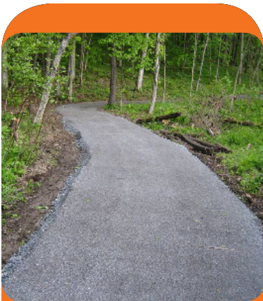
Shaver's Creek Environmental Center Centre County
