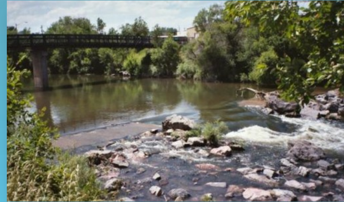
Sanitary Sewer Crossing
