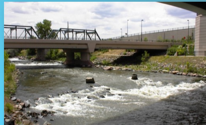
Stabilization Drop Structure
