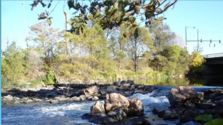
Sheet Pile Check Dam
