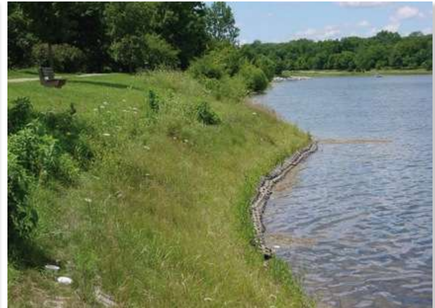
Same site with fully vegetated concrete block/geotextile installation completed
