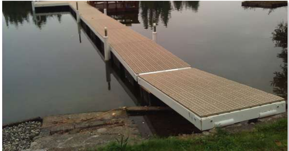
Galvanized steel frame floating dock with marine-grade PVC. No toxic chemicals are in this recyclable decking.
