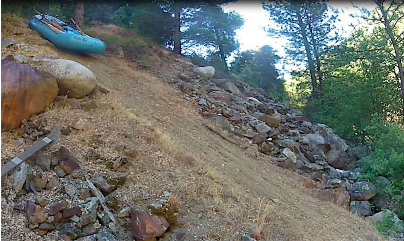
Tuolumne River launch: too steep for boats, people, and is causing erosion and bank destabilization
