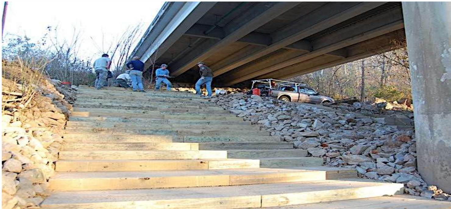
Staircase launch adjacent to bridge on the Harpeth State Scenic River in Tennessee
