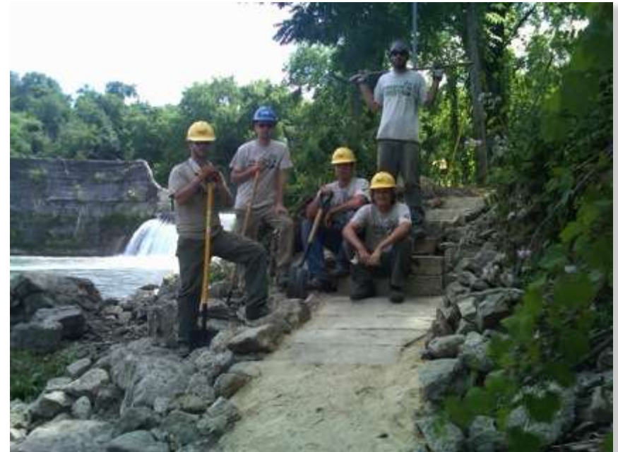
Example of pre-molded concrete slabs for steps using rocks found on site
