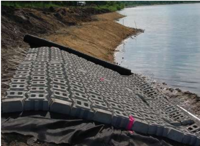
Articulating concrete block installation with geotextile fabric
