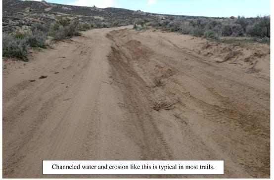
potential for severe erosion. A perfect example of this is the Play Area and the trail leading into it. Water from far up on the hill is trapped in the deep eroded cup of the trail and play area so all the water and sediment drains into the main staging area instead of off to the sides in the natural drainage courses.
