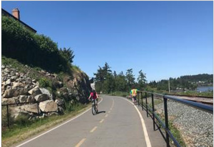
The E&N Rail Trail Humpback Connector on near Victoria, British Columbia. (Photo courtesy of Capital Regional District)
