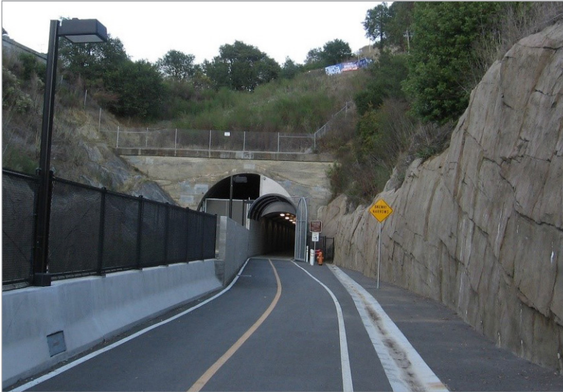
The shared-use Cal Park Hill Tunnel along the SMART commuter rail line in California (Photo courtesy of the Marin Independent Journal)
