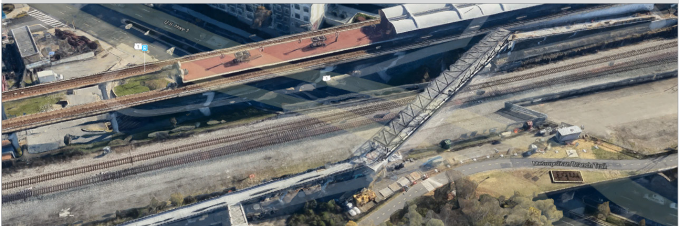
Metropolitan Branch Trail in Washington DC, with bridge over railroad connecting Metro station to trail. (Photo courtesy of Google)
