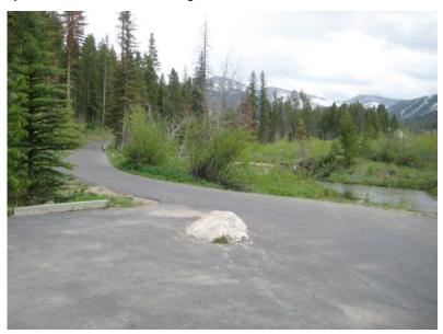
impaired trail users. In this case, desirable goals for universal access must be balanced with some trail user's perception that wide, concrete and asphalt trails detract from the natural beauty of the area. The drastically rising costs of asphalt and concrete must also be considered and balanced when determining if a trail should be constructed with these products to accommodate mobility-impaired users.
