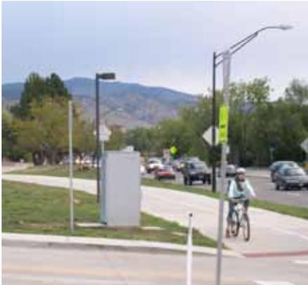
**Sidepath Separation.** On a multi-lane road, sidepath maintains an appropriate separation from 45 mph arterial. At intersection, the path moves toward the roadway edge for maximum visibility.
