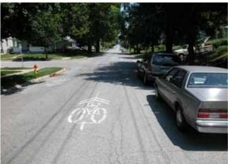
Shared Roadways. Top: Parking lot is defined with a white stripe and a shared lane marking is used to indicate presence of bicycles and position cyclists away from door zone. Bottom: Use of shared lane marking (sharrow) to indicate continuous route and position cyclists on a low-volume street. (Burt Street, Omaha, Nebraska)
