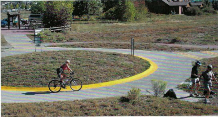
A "bicycle roundabout" on the heavily-used Mary Carter Greenway Trail in Littleton, Colorado
