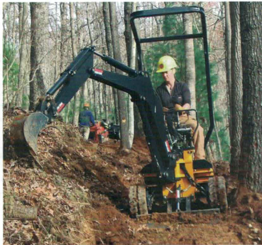
Microexcavator: small machines have big potential for building and maintaining trails
