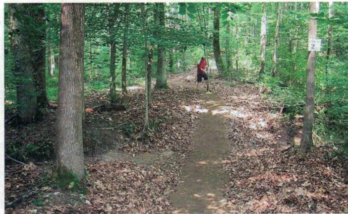
AFTER: creating a dry and durable trail surface
