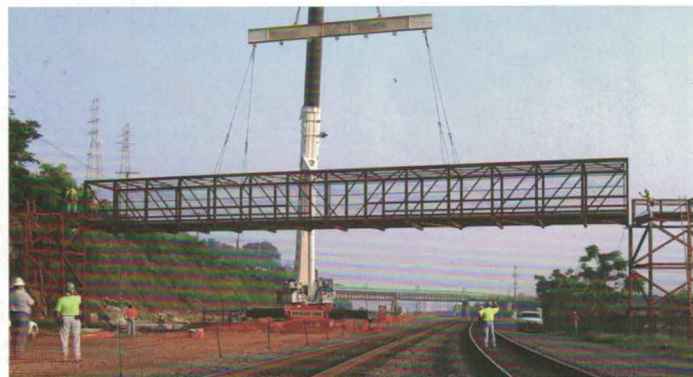
New trail bridge over the railroad (photo by Mary Shaw)
