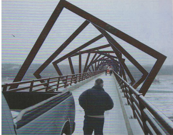
Steel "cribbing" is all part of the integrated artistic experience of the bridge (photo by Snyder and Associates)
