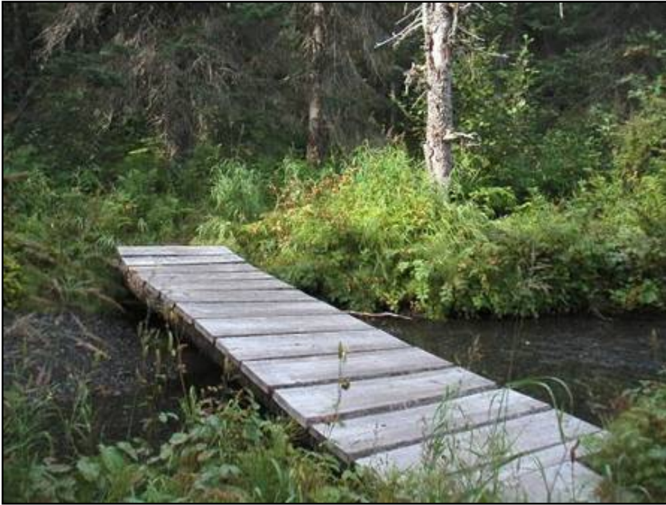
Structure has all the basic structural elements and is over actively flowing water.
