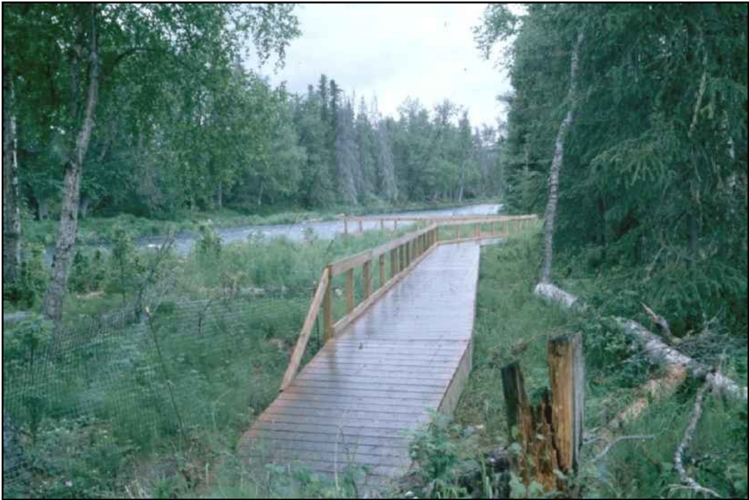
Elevated trail structure with multiple pilings and has handrails.
