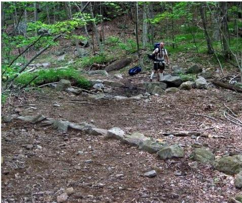
Figure 2. Sustainable tread grade-reversals (top) are 100% effective in draining water and rarely require maintenance. Drainage ditches (middle) are easily installed, with excavated soil mounded just downhill, but require annual cleaning to maintain their efficacy. Water bars constructed of rock (bottom) or wood are longer lasting but also require cleaning and are generally not tire friendly.
