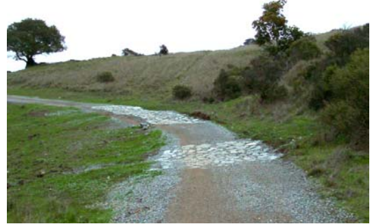
FIGURE 13: ARMORED DRAINAGE DIPS AT CHINA CAMP STATE PARK
