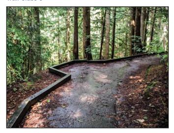
**Trail Class 5: Tread**—The tread is wide, firm, stable, and generally uniform. Trails are commonly hardened with asphalt or other imported material.
