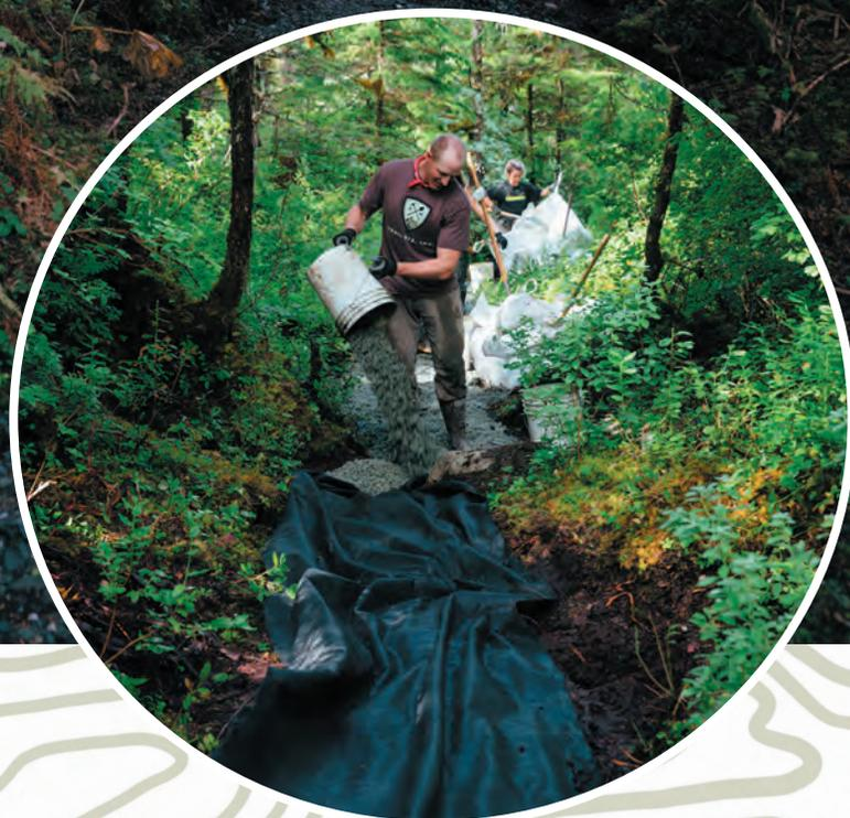
CCC Crew members lay new gravel on top of tarp to prevent the smaller gravel grain from getting washed out.
