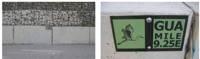
Wall-mounted signs were adhered to a flood wall because obstructions were not permitted within a flood control channel.
