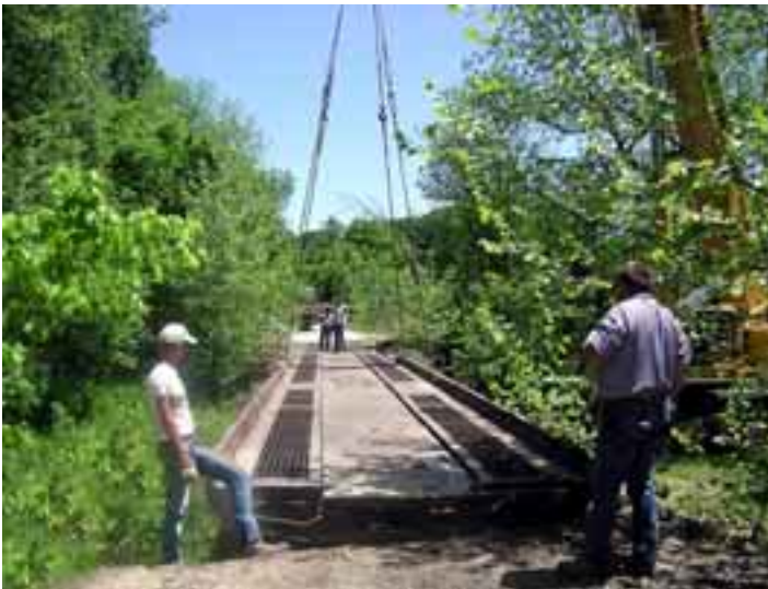
Placing the flatcar bridge (photo: Ozark Greenways)
