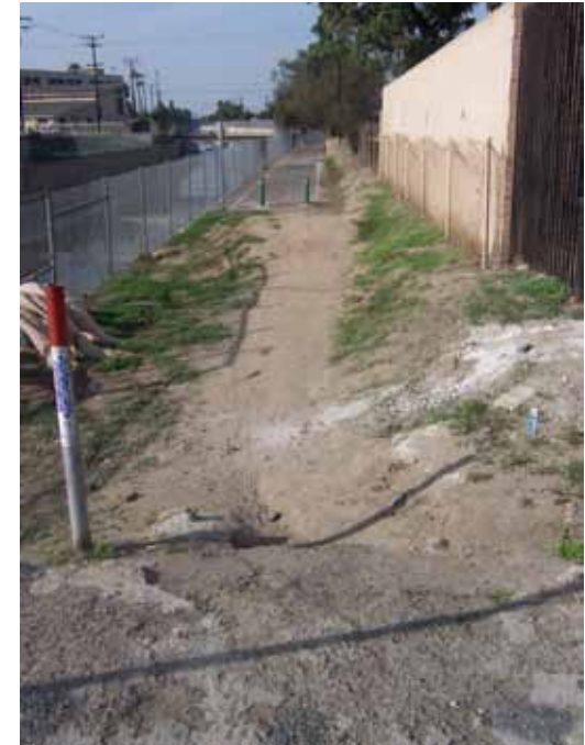
A 50-foot section of unpaved path north of Rosecrans.
