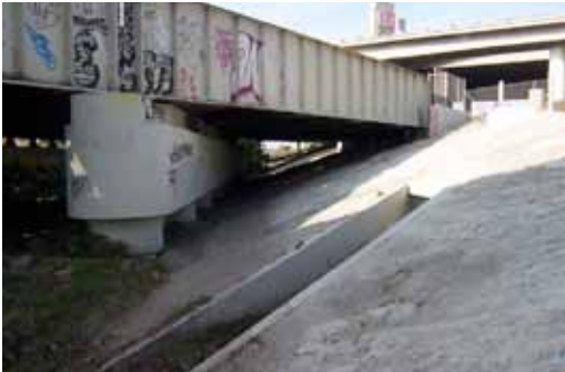
Storm drains and the Alameda corridor rail lines dictate the likely connection between the city and county portions will need to be in the channel.
