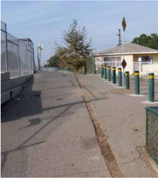
Shallow trench in trail is a hazard for cyclists.
