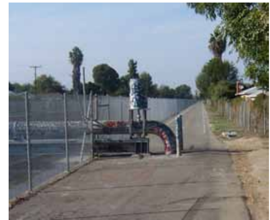
Pipe projecting into trail north of Washington Elementary.
