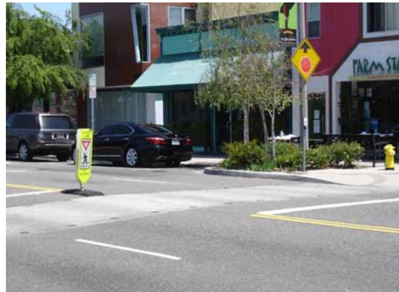
Curb extensions, in-pavement flashers and R1-6 in-roadway signs help improve safety at this crossing.
