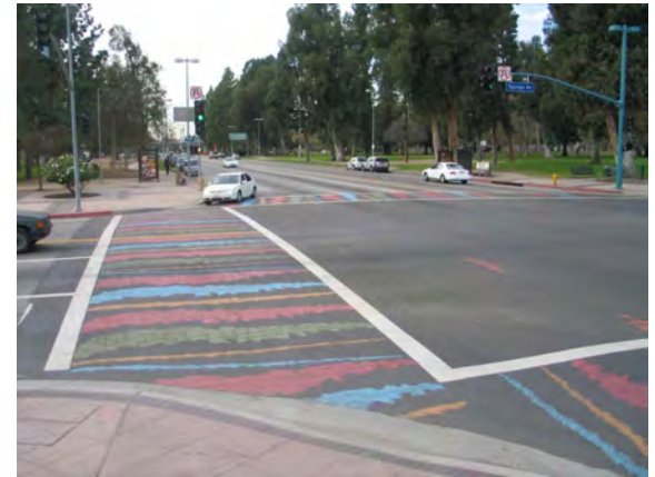
Applications of thermoplastic crosswalk markings Source: Integrated Paving Concepts
