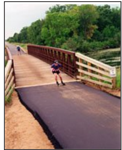
The surface of a trail can help determine its target markets. In-line skating requires smooth paved surfaces and well-maintained bridge crossings. Here, on the Paul Bunyan Trail in Minnesota, in-line skaters share the trail with bicyclists. In the winter this trail is used by snowmobilers (non-studded treads only) and cross-country skiers.
