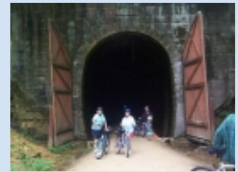
A view of the entrance to one of the Elroy-Sparta Trail's landmark train tunnels.
