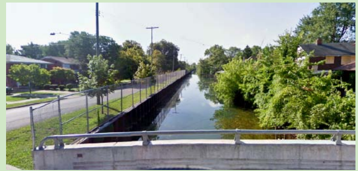
Fox Creek Channel Adjacent to Alter Road (Source: Google)
