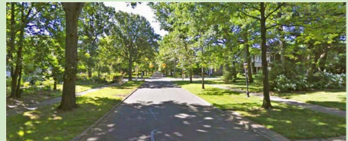
Typical Condition Along Burns Street (Source: Google)
