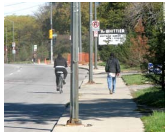
Street with No Bike Facilities and Few Pedestrian Amenities (Source: JJR)
