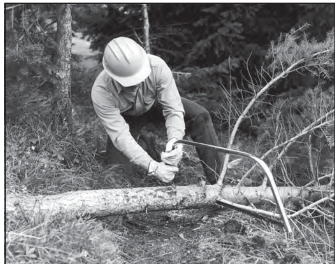
Bow saws effectively clear trails.
