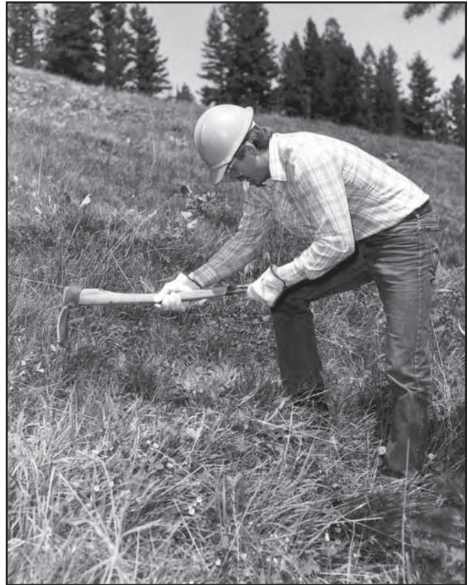
Grub hoe being used for trail work.
