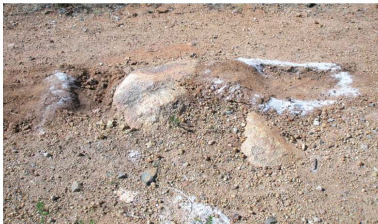
Figure 5: Trail surface modified to create a TTF in John Forrest National Park, Western Australia: note the end of the feature has been reinforced by cement
