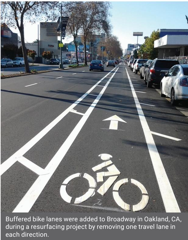
Buffered bike lanes were added to Broadway in Oakland, CA, during a resurfacing project by removing one travel lane in each direction.
