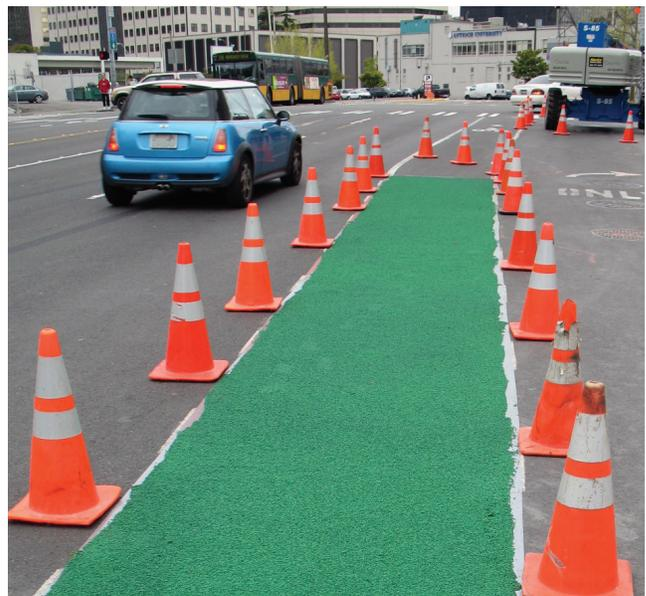
A marking plan is essential to ensure bikeways are marked as intended following a resurfacing. Green pavement markings have received interim approval from FHWA, but agencies must seek approval from FHWA prior to using green markings.
