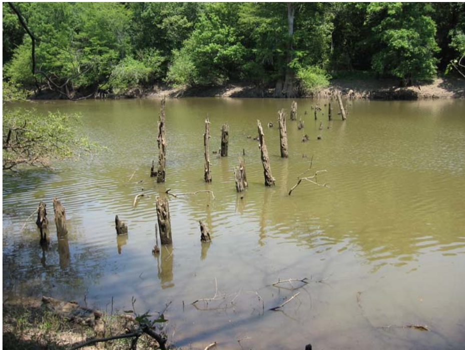
Figure 27: Rock Roe Bridge site showing wooden bridge piers. View is from the west bank of the bayou, towards the east.
