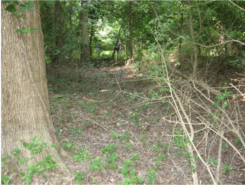
Figure 34: The definition of the roadbed has been eroded significantly since it was last used in the early 20 th century.
