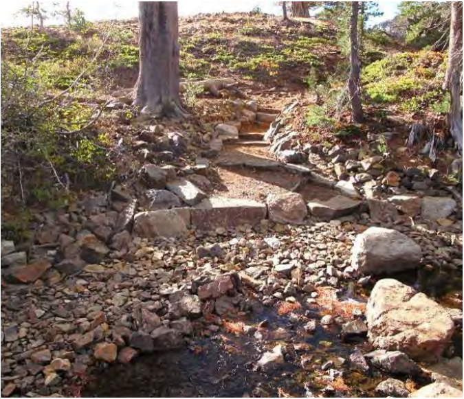
Figure 4–13. Bank armoring in the approach to a shallow stream ford. Lake Tahoe Basin Management Unit, California. USDA photo by Garrett Villanueva.
