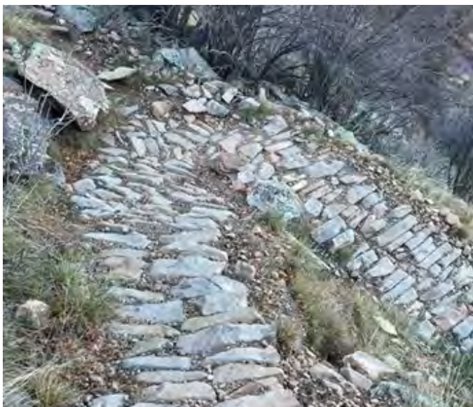
Figure 4–56. Rock pitching used to protect a steep section of trail. Grand Canyon National Park, Arizona. USDA photo by Kerry Wood.
