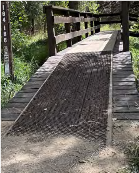
Figure 4–23. Trail bridge approaches should climb at a 2– to 8–percent grade or be a step(s) that climbs to the level of the bridge deck. Carson National Forest, New Mexico. USDA photo by Kerry Wood.
