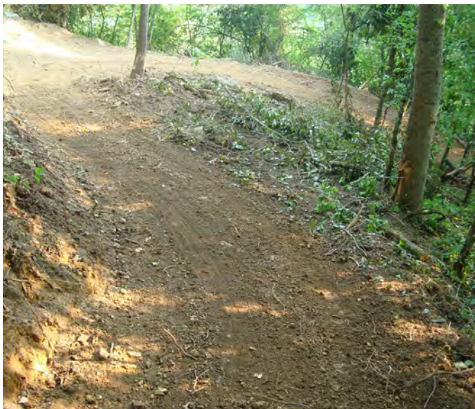
Figure 4–30. Use natural obstacles, like the tree at the top of this photo, as guide structures to prevent shortcutting. Wayne National Forest, Ohio. USDA photo by Scott Johnson.
