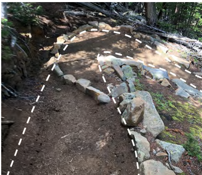
Figure 4–33. Rocks on the inside of the turn help prevent crosscutting the switchback. Rocks in the tread provide inside drainage before the turn. Pike–San Isabel National Forests, Colorado. USDA photo by Adam Carroll.
