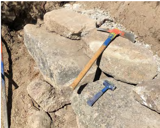
Figure 4–40. Use smaller rock to backfill and compact behind the larger rocks to stabilize the rock wall. Pike–San Isabel National Forests, Colorado. USDA photo by Adam Carroll.
