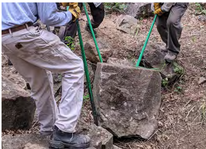
Figure 3–19. Rock bar and fulcrum used to move a large rock. Cibola National Forest, New Mexico. USDA photo by Kerry Wood.
