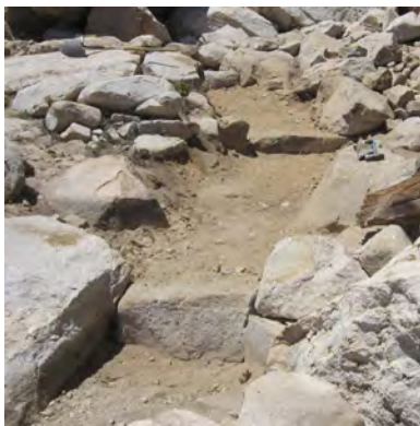
Figure 2–15. A developed (class 3) trail has a consistent tread and less-frequent obstacles; imported materials may be present. Inyo National Forest, California. USDA photo by Jess May.
