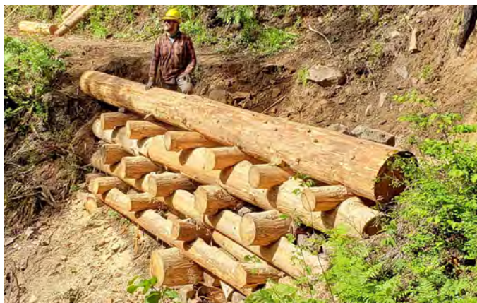
Figure 4–41. Where no large rocks are available, log crib walls may be a viable solution. Columbia River Gorge, Oregon. USDA photo by Nathaniel Brodie.
