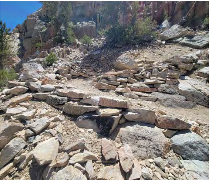
Figure 4–35. Modified climbing turn with rock retaining walls on the upper and lower legs. Inyo National Forest, California. USDA photo by Jess May.
