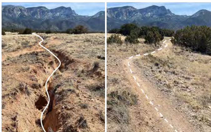
Figure 2–1. The deeply rutted and abandoned trail on the left (solid line) was built without physical sustainability principles in mind. The trail on the right (dotted line) is nearby and is well-located on a hillside at an average grade appropriate for the prevailing hillside slope and with frequent grade reversals. Cibola National Forest, New Mexico. USDA photo by Kerry Wood.
