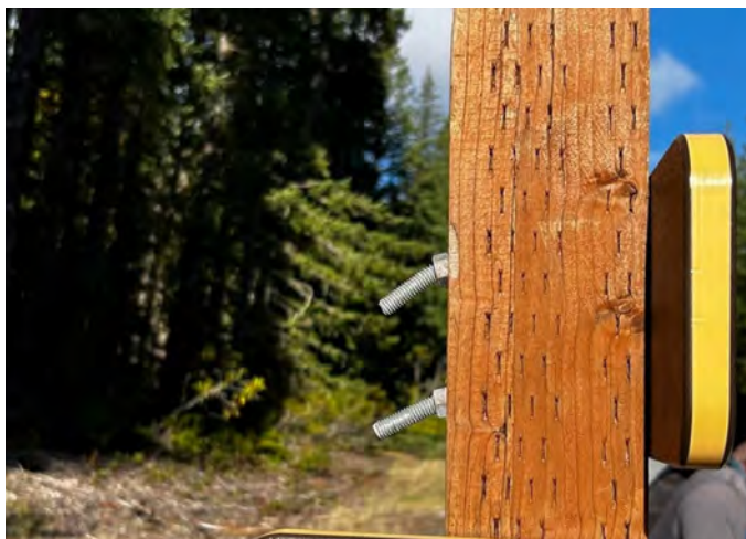
Figure 3–1. Bending the ends of through bolts can help prevent sign theft. Mt. Hood National Forest, Oregon. USDA photo by Meckenzie Helmandollar-Powell.
