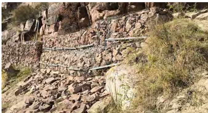
Figure 4–45. Gabion retaining structure. Ashley National Forest, Utah. USDA photo by Nathan Emer.
