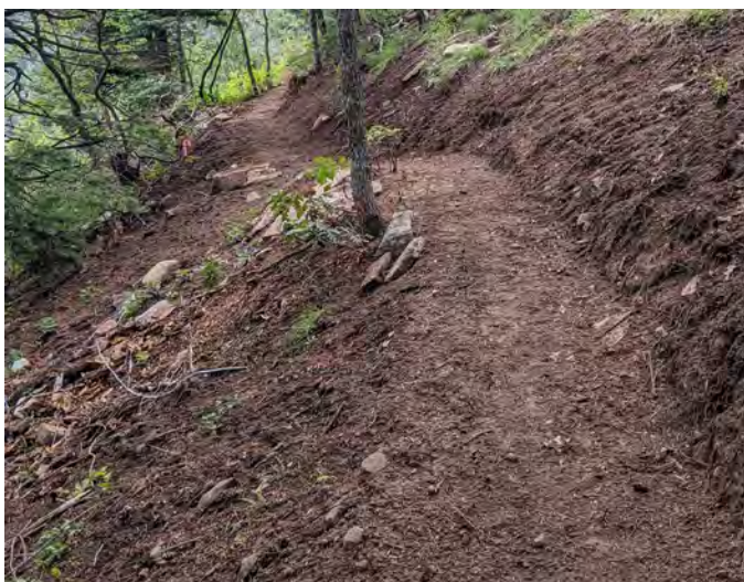
Figure 6–8. Enhance the user’s experience and improve drainage using grade reversals by going above trees and rocks. Cibola National Forest, New Mexico. Courtesy photo by Jenny Blackmore.
