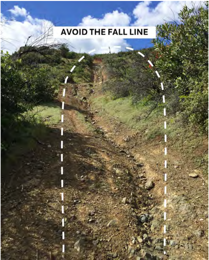
Figure 2–22. Avoid routing trails parallel to the fall line. Fall line trails easily erode, are expensive to repair, and often cause environmental damage. Las Padres National Forest, California. USDA photo by Scott Johnson.
