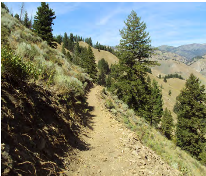
Figure 6–12. A sidehill trail that is being made more physically sustainable by excavating the backslope. Note the bushes encroaching on the trail in the background. Boise National Forest, Idaho. USDA photo by Scott Johnson.
