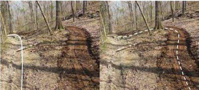
Figure 4–5. The old trail (solid line) was realigned uphill (dotted line) to create a grade reversal. Tennessee. USDA photo by Scott Johnson.
