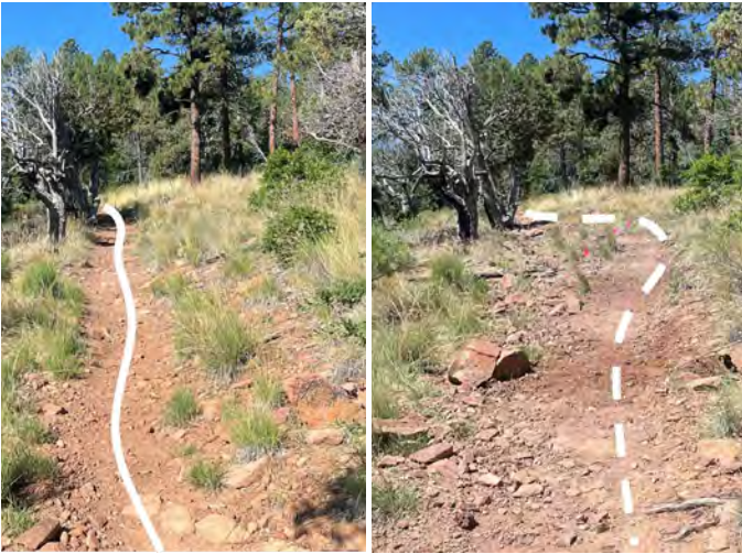
Figure 4–4. On the right, a minor realignment uphill of an existing trail to create a grade reversal, also referred to as a forced uphill undulation. Cibola National Forest, New Mexico. USDA photo by Kerry Wood.
