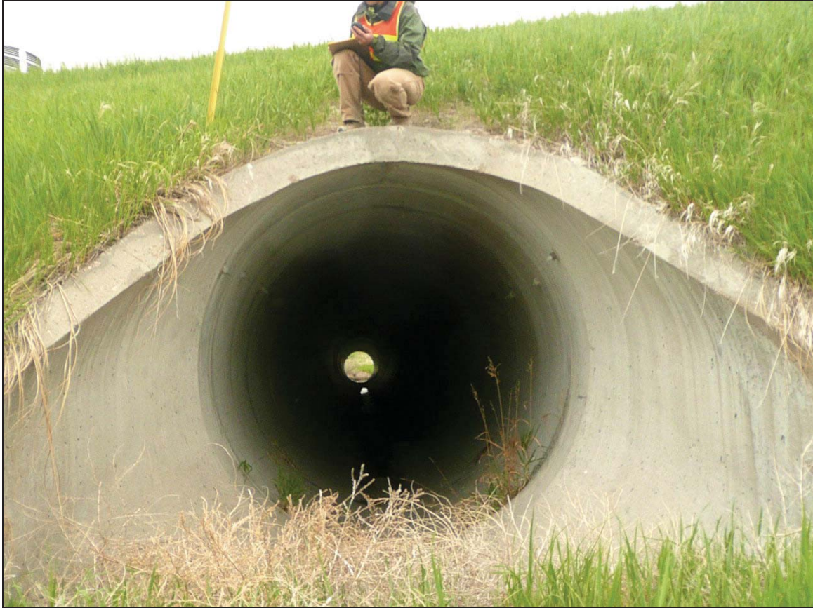
Figure 50. Photo. Continuous wildlife underpass on divided highway (Credit: Tony Clevenger).
