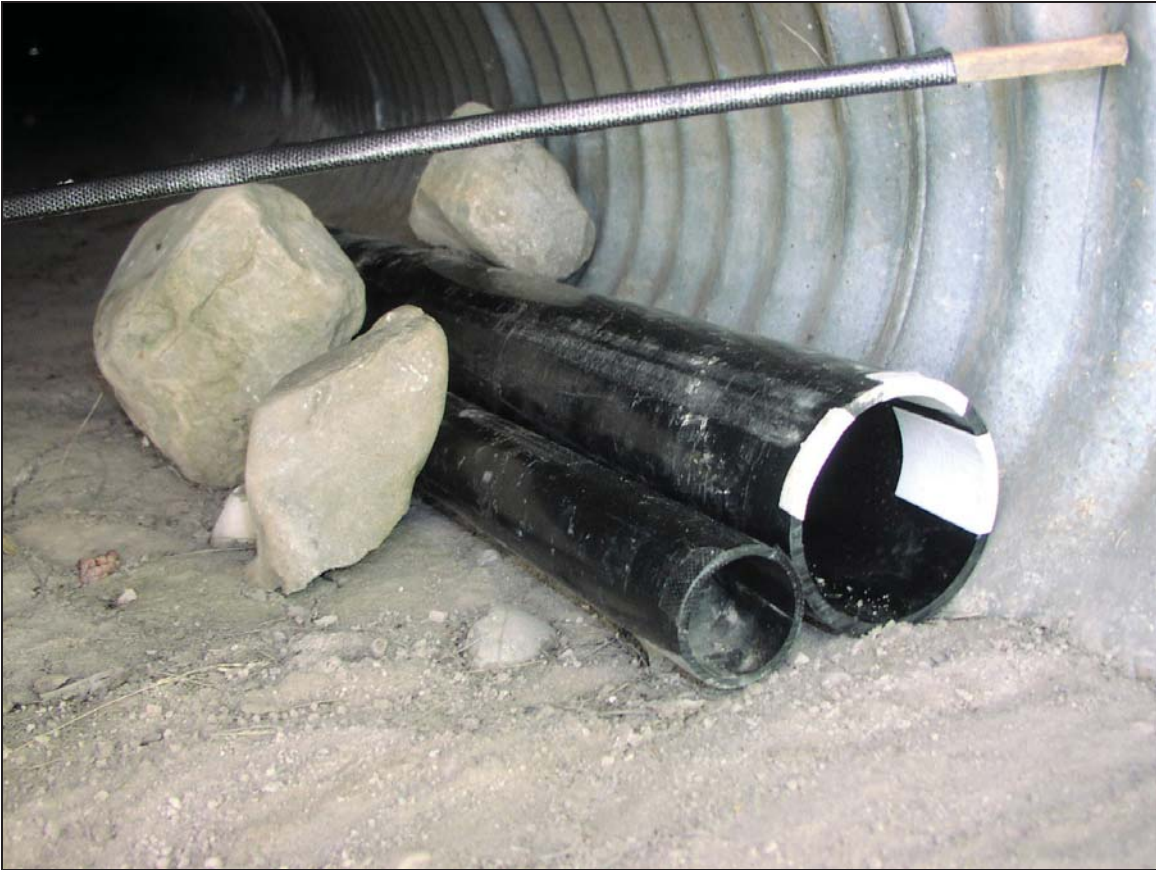
Figure 48. Photo. Pipes placed in culverts to provide cover for small mammal movement (Credit: Tony Clevenger).
