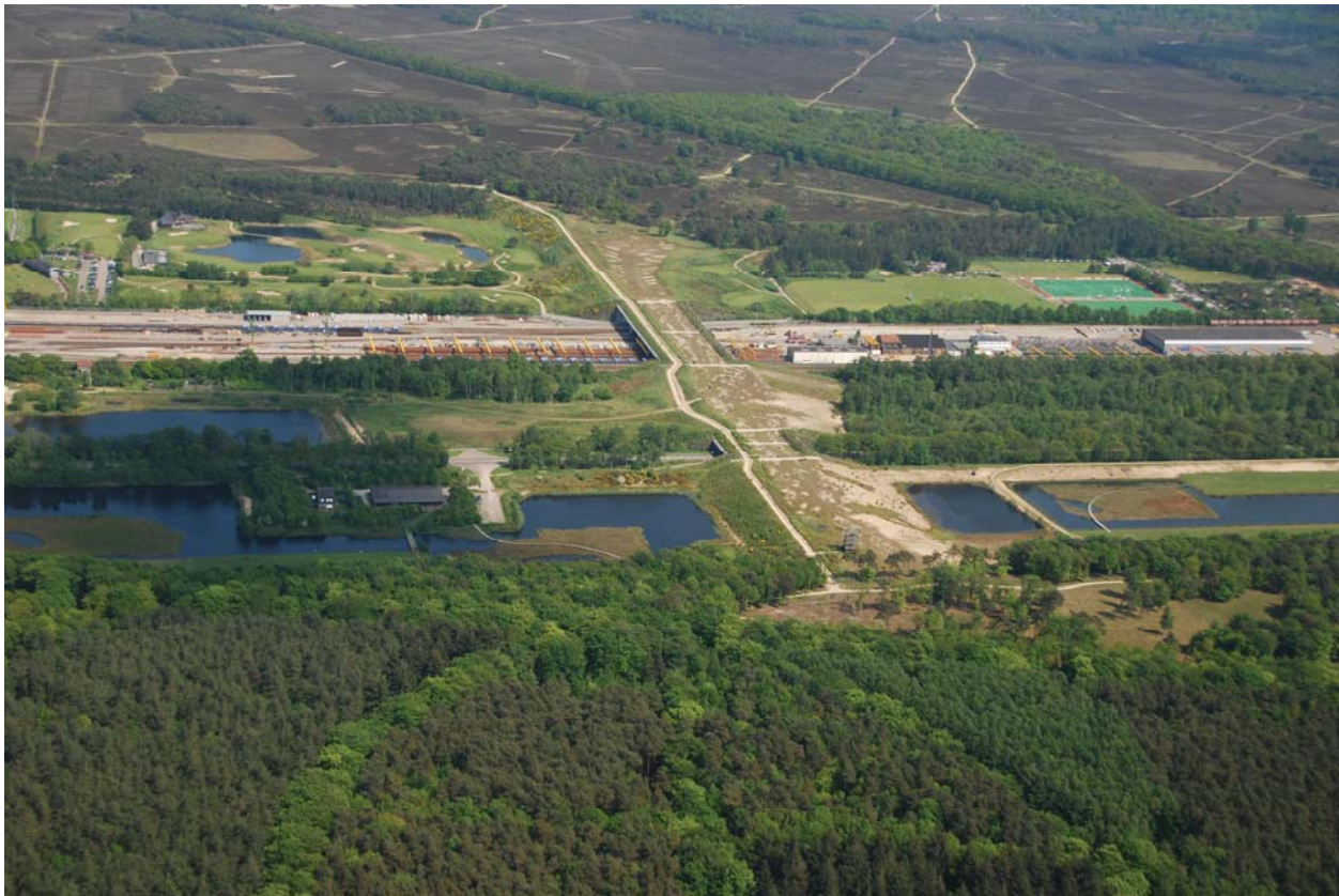
Figure 27. Photo. Most wildlife overpasses or landscape bridges are less than 70-80 m long; however, the one shown above near Hilversum, The Netherlands, is 800 m long and spans two roads and a railroad. (Credit: Goois Natuurreservaat, The Netherlands/Photo: W. Metz).
