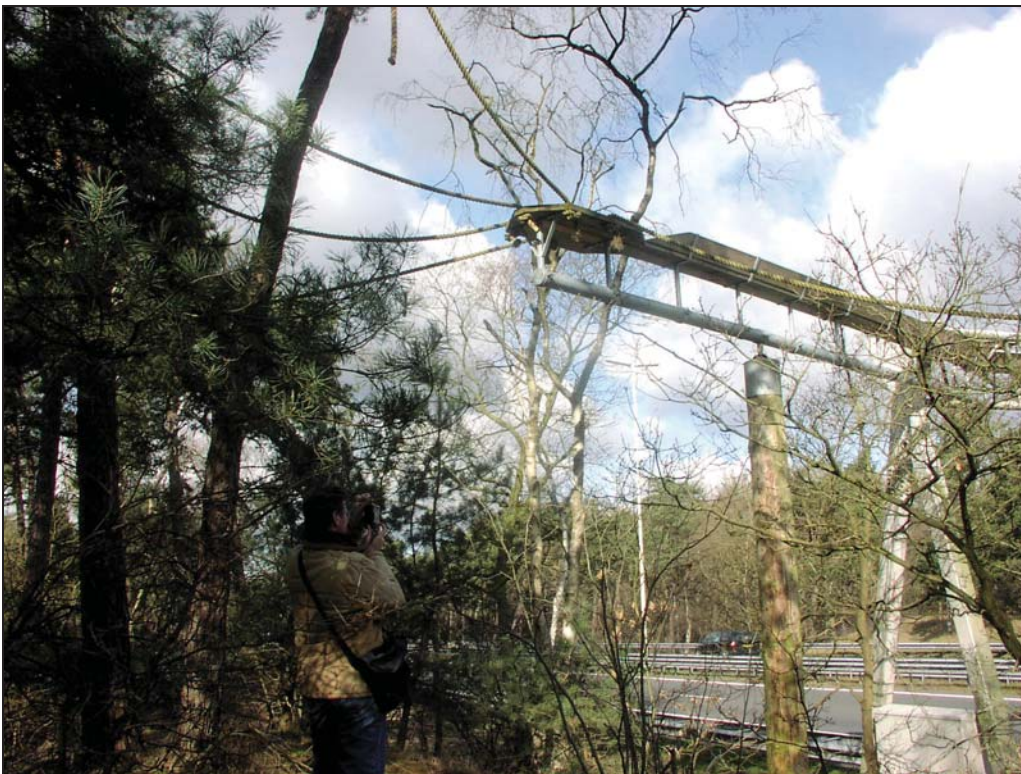
Figure 38. Photo. Ropes extending out from canopy crossing to forest canopy (Credit: Tony Clevenger).
