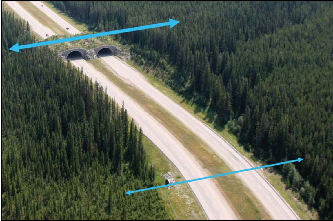
Figure 28. Photo. Crossing structures are site-specific movement corridors that link wildlife habitat separated by pavement and high-speed vehicles (Credit: Jeff Stetz).
