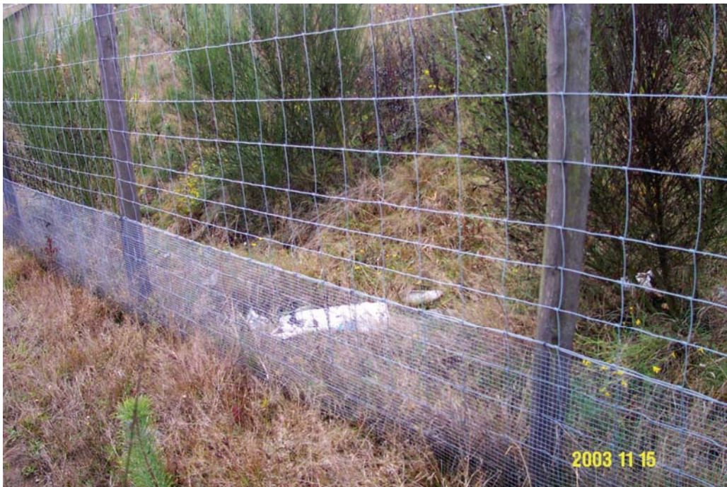
Figure 70. Photo. Small and medium-sized mammal fence material spliced to large mammal fence material (Credit: Nancy Newhouse).
