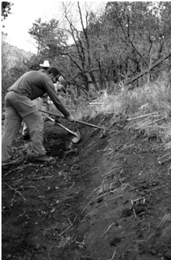
Backslope work on a trail.
