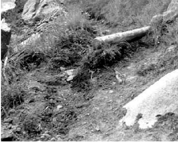
Maintenance tasks take a variety of shapes and pose their own individual challenges. Too much water and sediment washed out this waterbar.
