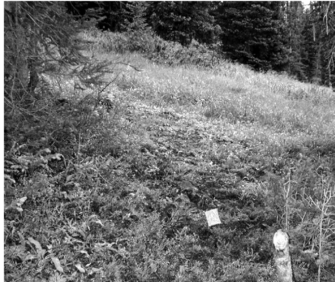
Pin flags are used to mark the center line of the planned trail tread.
