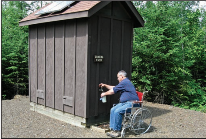
Figure 18—The water pump inside the pumphouse at Vermilion Falls Recreation Area on the Superior National Forest is powered by the solar panels on the roof. People can obtain drinking water without using a handpump at this site that has no electric service.
