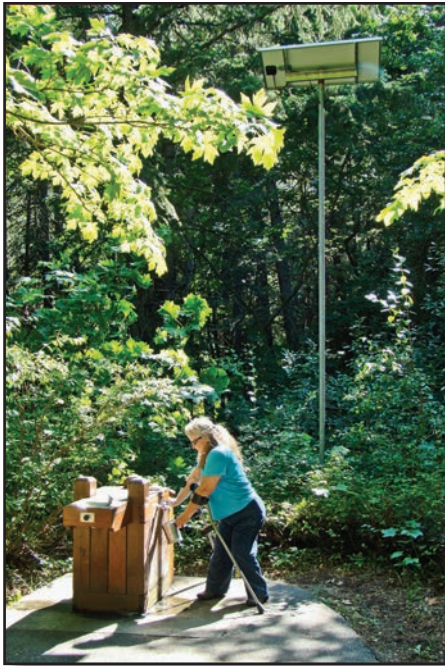
Figure 103—Solar water pumps and batteries can be housed in small pedestal enclosures and powered by solar panels on an adjacent pole.
