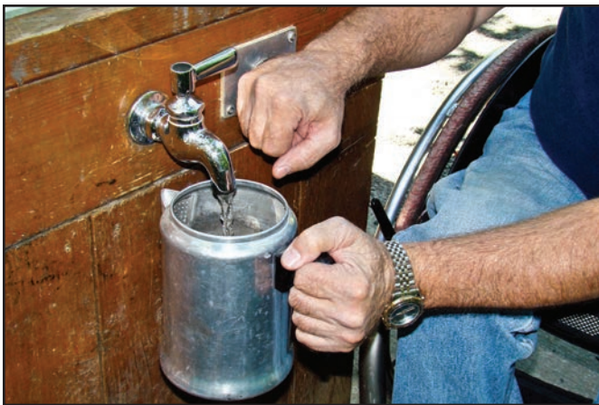
Figure 104—A solar pump provides pressure for this water spigot. A camper uses accessible controls to fill his coffee pot.
