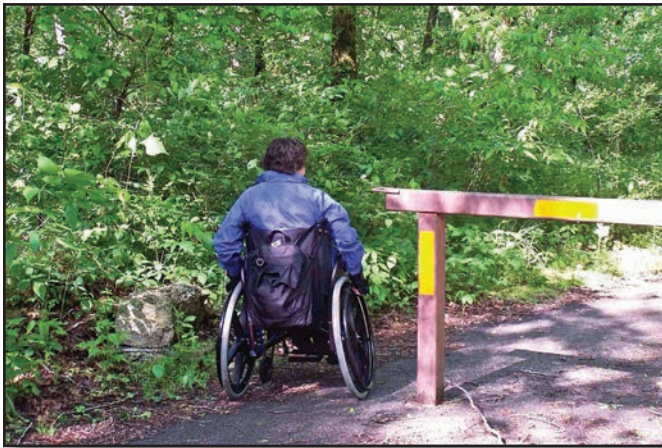
Figure 22—One way to get around a vehicle road closure gate: a paved bypass.
