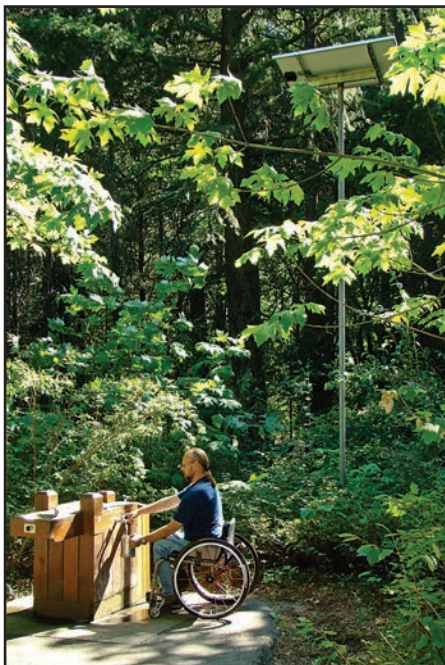
Figure 19—The water pumps for many campgrounds, such as this campground in the deep, narrow Icicle River Valley of the Okanogan-Wenatchee National Forest, can be housed in small pedestal enclosures and powered by solar panels on an adjacent pole. The pedestal enclosure also houses solar batteries.
