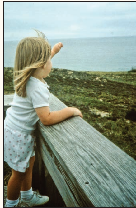
Figure 67—Caution: Railings with horizontal rails make an inviting ladder for small children.
