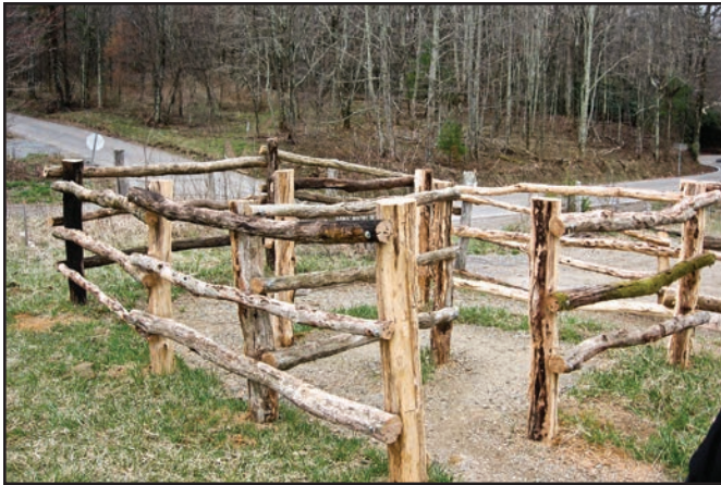
Figure 47—The winding configuration of this rustic chicane where the Appalachian Trail crosses Tennessee Highway 91 and the Osborne farm allows pedestrians to pass through the fence to use the trail but keeps motorized users out and horses inside the farm fence.
