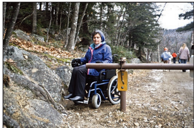
Figure 21—This road closure gate does not provide enough clearance to allow pedestrian passage.
