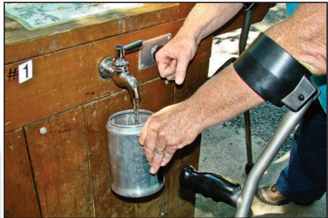
Figure 20—This water spigot is operated by first pushing the handle to one side, then pressing the push button. The water will stop when the button is no longer depressed.
